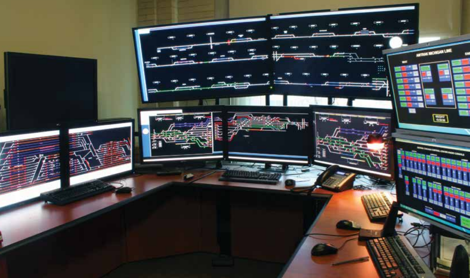
▲ Work once performed at two towers is now performed in the Union Station dispatching center, shown May 22, 2017. Station tracks are displayed on the two monitors on the left; screens on the center desk cover Chicago yard movements and the approach to the station in New Orleans. On top is Amtrak's Michigan line between Porter, Ind., and Dearborn, Mich. Two photos, Bob Johnston
