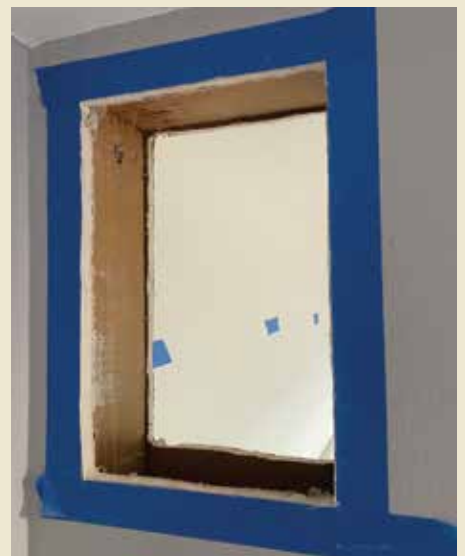
Fig. 4. Don had to treat the adjacent closet as a tunnel; so, he had to cut entrance and exit "portals" into the drywall. After he had made a large hole, he used a hacksaw with an extra-fine blade to finish the task.
