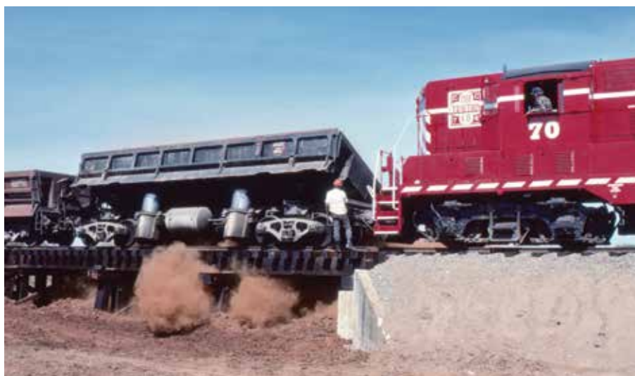
Top: Engineer J.M. Jackson watches from the cab of GP7 70 as ATSF air dump hoppers are emptied at Willow Creek, the Bridge 26 fill project. Roadmaster Howard Menking oversaw the filling and strengthening of at least four additional trestles, including this one, following the 1973 collapse at Dry Creek. Above: A B&B worker pulls the trigger on a Santa Fe air dump at Willow Creek, north of Herald at milepost 26. This fill project was one of several during the decade.
