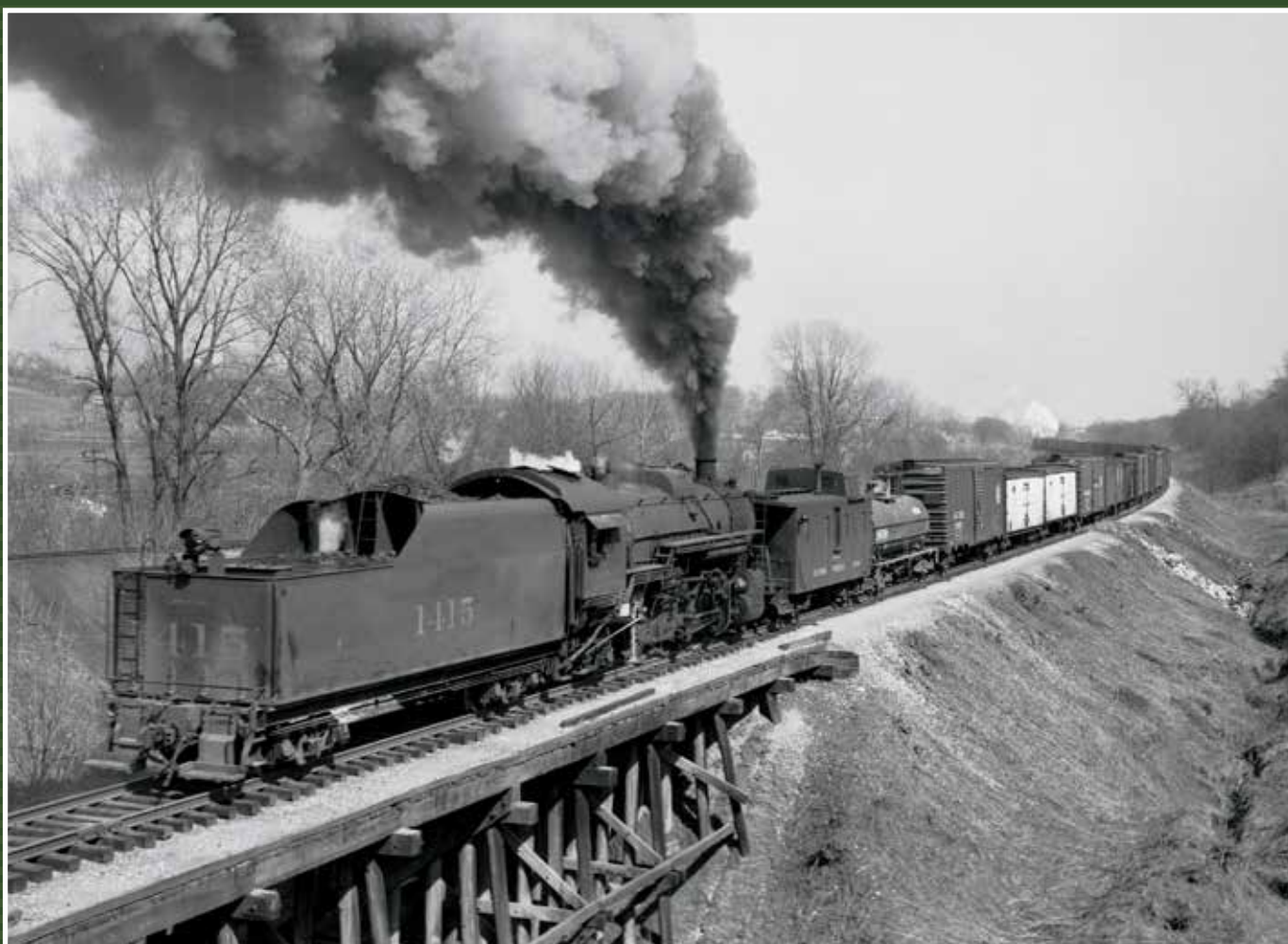
Smoking No. 1415 pushes train 81 across a wood trestle on May 5, 1950, at Church, Ill., southeast of East St. Louis.
