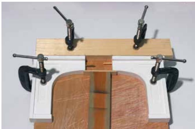
2 Small rods are added to form reinforcement bars to secure the new section of plaster.
