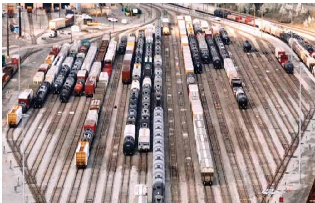
▲ Reconfiguration of the Cumberland, Md., yard — which had its hump shut down in 2017 — included removing the hump and adding new switching leads and an additional classification track. The changes have allowed CSX to bring back trains that had been assigned to smaller facilities. CSX
