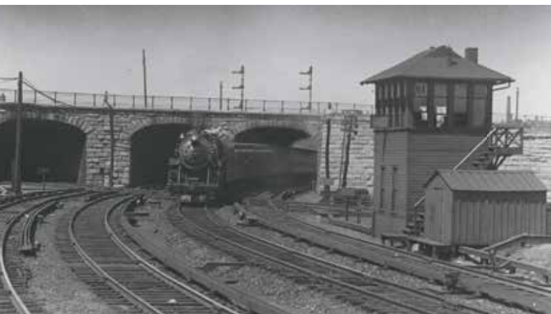
▲ Increasing clearance at the North Avenue viaduct, shown circa 1943, is a challenge because the B&P Tunnel is immediately below, and the area now includes light rail and more roadways. Trains collection
