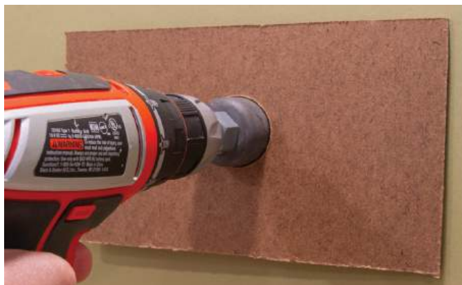
③ Jim used a 1½" hole saw to cut the opening for the cap. He applied silicone caulk from the back to glue it to the fascia.
