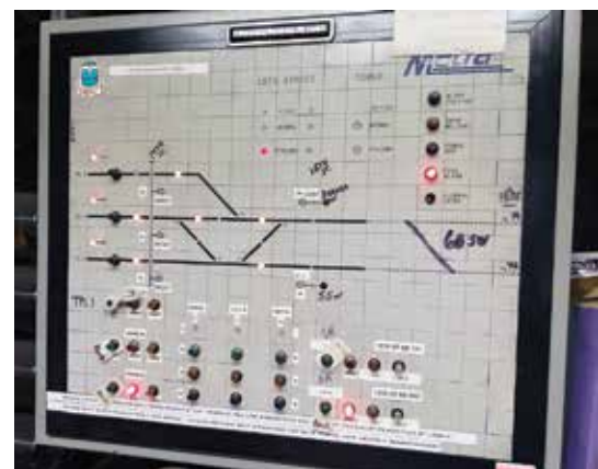
▲ The model board shows the relatively simple crossing the tower controlled at its closure, a far cry from the five-way, multi-main junction at its birth.
