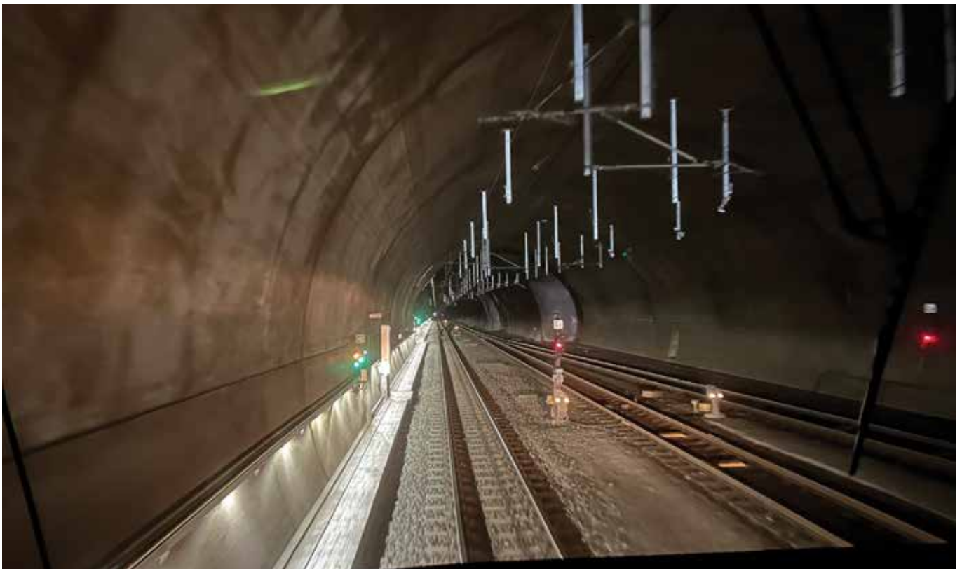
The locomotive driver's view as an auto-transport train bound for Sagliains begins its trip through the mostly single-track Vereina tunnel. A trip through the 19.1-kilometer (11.9-mile) tunnel takes about 18 minutes. Drivers and passengers stay in their cars for the trip.
