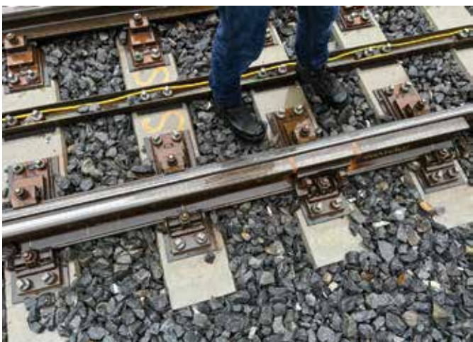
Another element of the design allowing the bridge to adjust to its changing environment: a section of the rail at the hillside end slides to accommodate movement.
