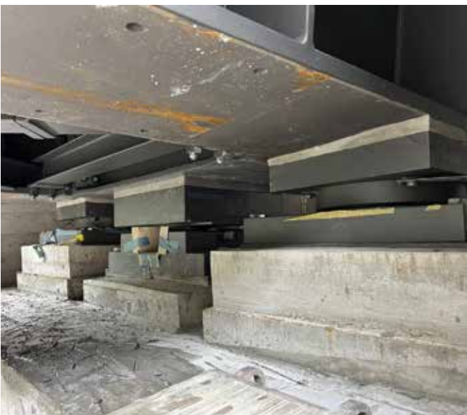
Underneath the bridge deck, these supports allow the deck to "float" enough to move along with the gradually sliding hillside at the west end of the 377-foot structure.
