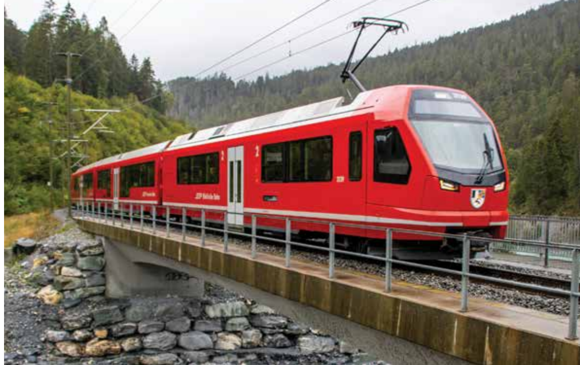
A train from Disentis/Mustér to Chur crosses the Carrera Creek bridge. The relatively nondescript structure, over a stream feeding the Rhine, is notable for the monitoring and warning systems it offers to address a history of flash flooding that has destroyed two earlier bridges in the same spot.
