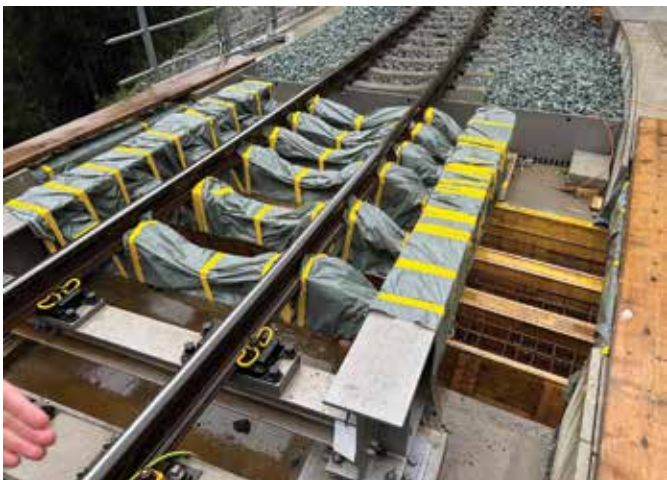
The sections wrapped in gray plastic are the removable pieces that allow the Castieler bridge's length to be adjusted to allow for the moving hillside that forced replacement of the previous structure.
