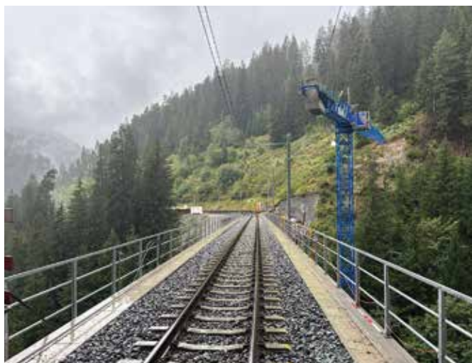
A view from the tunnel mouth of the Castieler Viaduct provides a look at the slowly sliding hillside. This side of the valley occupied by the rail line is sliding from 2 to 10 centimeters per year — as much as 4 inches — making the line the railway’s most expensive to maintain.
