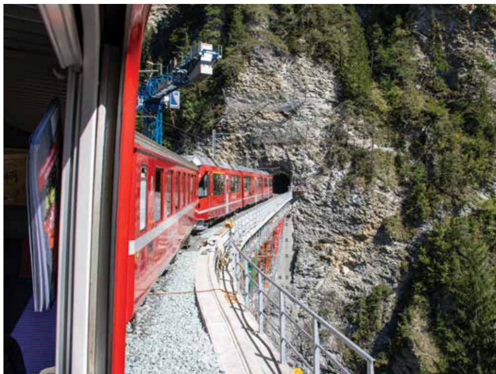
Much of the railroad’s older equipment still features windows that open, a boon for photography that made possible this shot of an Arosa-bound train crossing the still-unfinished Castieler Viaduct on Sept. 10, 2024. The hillside on the tunnel end provides a stable anchor for the bridge, unlike the other end.
