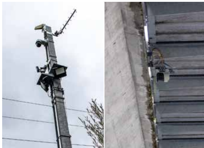
Monitoring for the Carrera Creek bridge includes a camera mounted on this pole on the creek's east side, as well as a device tucked under the bridge that tracks the water level through a cellphone app.
