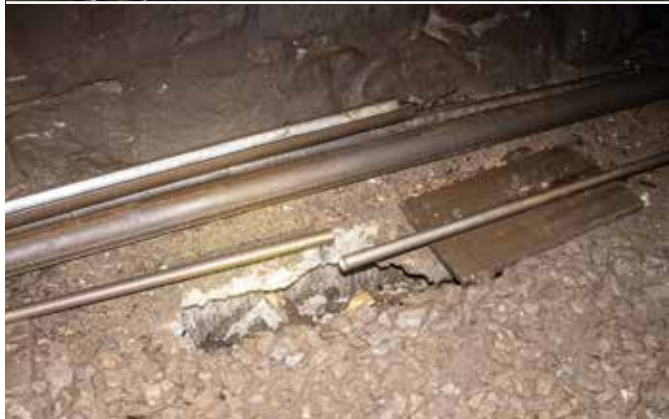
Top: With tracks and catenary removed, the arrow-straight, 3.6-mile original Albula tunnel is now in the process of being turned into an emergency access road. Below: A portion of the tunnel's drainage system has collapsed, leaving a hole in the floor.
