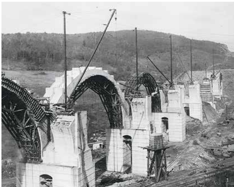
Three arches and six piers of the Martins Creek Viaduct during construction on Aug. 19, 1913. Steel falsework was used to support the concrete forms. University of Washington
