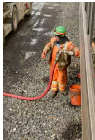
▲ Fueling at Chapleau is a requirement in each direction. Here, each of the RDCs gets about 420 gallons on the west-bound trip.
