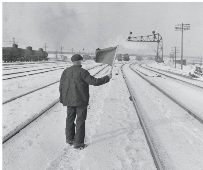
Jack Delano, an Office of War Information photographer, captured this January 1943 image of an Indiana Harbor Belt flagman carrying out Rule 99. Using cardstock flagmen on our layouts is a practical way to observe the rule. Photo courtesy of the Library of Congress
