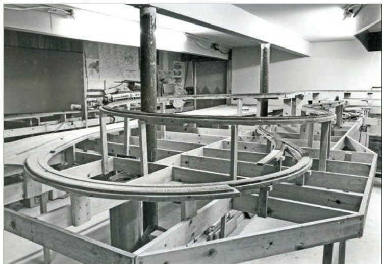
Photos dating to the early 1970s show the template I drew on kraft-paper on the floor from my \frac{3}{4} "-scale Allegheny Midland track plan; the first 1 x 4 benchwork; the long kraft-paper template partially unrolled on the benchwork; an optimistic me checking a tunnel portal position; and a view of the peninsula showing the standard 40" benchwork height. Track elevations ranged from 43" to 58", but I kept the benchwork top surface at 40" to allow the paper templates to be unrolled atop the benchwork as a final check on track positioning, reach-in distances, viewing angles, and other features.
