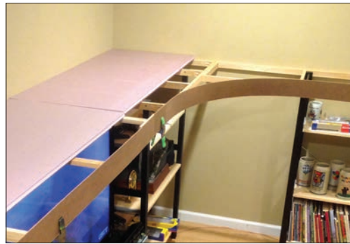
For the HO Port of Los Angeles, Bernie Kempinski used an open-grid frame made from 1 x 2 pine with 2" pink foam for the flat terrain. He found some dips in the foam and in the future plans to use a layer of 1/4" plywood on top of the foam to provide a flatter surface. All: Bernie Kempinski
