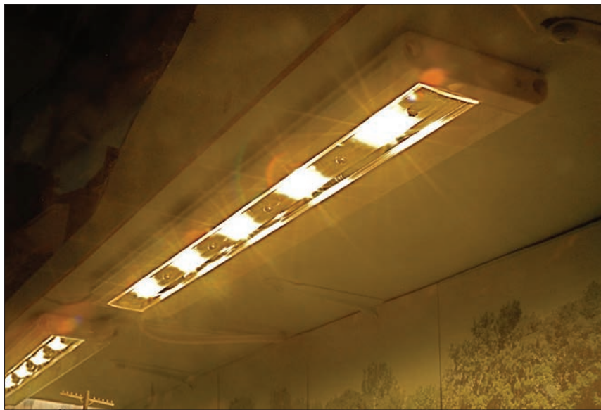
A commercial LED fixture intended for under-cabinet use produces a reddish (around 3200K) light. Moreover, when the LEDs are less than several feet above the track, as shown here, each LED head may create a distracting streak of light across the rails. In my experience, diffusers don't help much, so I suggest testing fixtures or strips of LEDs before buying them in quantity.
