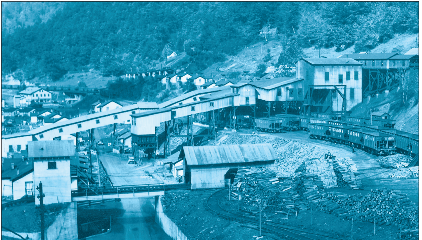
The West Virginia coal district accounted for more than 86 percent of the Virginian's freight. This sprawling coal tipples dominates the little mining town of Slab Fork, W. Va.
