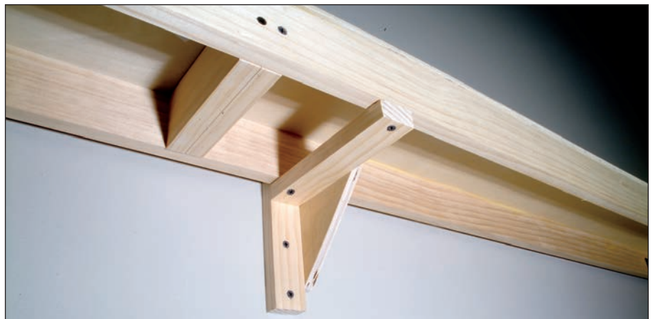
Simple homemade or commercial shelf brackets can support wall-mounted benchwork—in this case a simple 1 x 3 frame.
