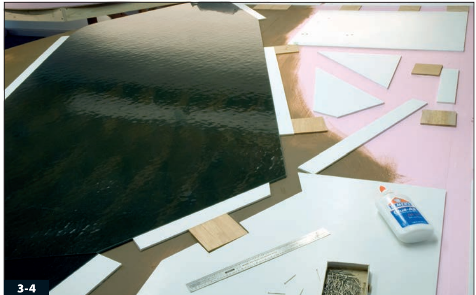
The square pieces of plywood serve as screw anchors. Similar pieces on the upper layer of foam provide a simple way to secure it. This makes it easy to remove if necessary. The upper layer of foam will sit on top of the glass, not beside it.
