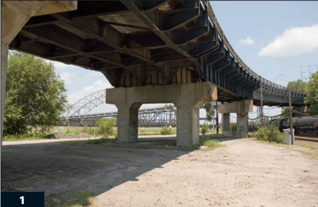
From a distance, this deck girder bridge appears to be curved.
