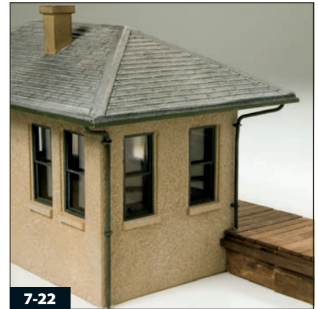
The downspouts add detail and cover the corner joints in the walls.
