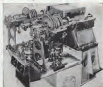
The Turbine for Union Pacific's New Steam-Electric Locomotive
