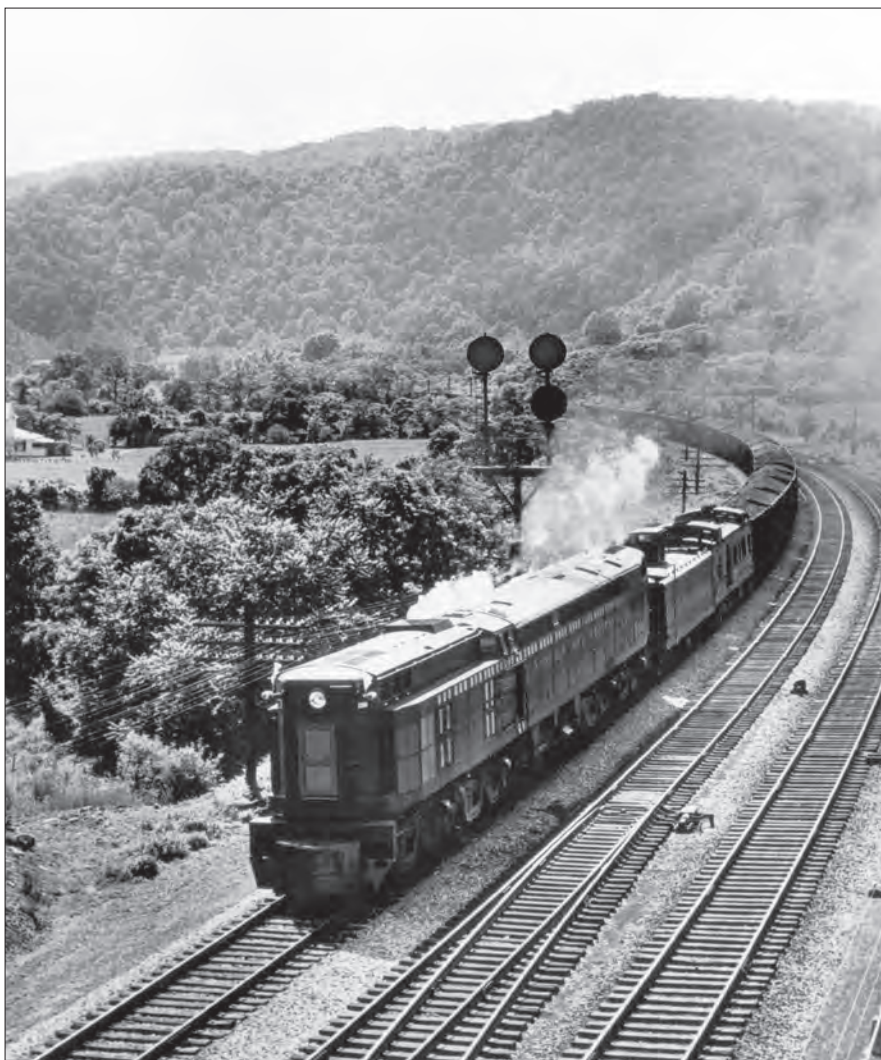
The TE-1 is pulling a dynamometer car and coal train on an early shakedown run in Elliston, Va., on June 2, 1954. Norfolk & Western Historical Society
