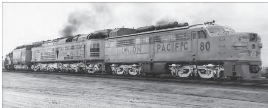
The lead unit of the coal-burning GTEL, shown in Council Bluffs, Iowa, in 1962, was a former Alco PA-1, which retained its 2,000 horsepower diesel engine. Lou Schmitz
