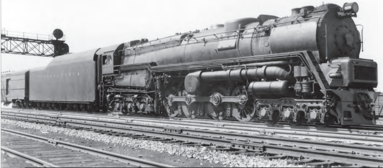
Pennsylvania RR No. 6200 sits in Chicago on July 15, 1945. It would run until 1949 before being scrapped. Visible on the right side is the 6,900 horsepower forward movement steam turbine. Note the massive steam line. PRRT&HS/The Keystone
