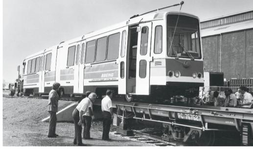
Boeing Vertol's first light rail vehicle, the first streetcar-type equipment built in the U.S. in more than 20 years, is loaded onto a flatcar at the company's plant in Philadelphia for shipment to Boston to begin testing. The cars proved to have short service lives. Boeing
