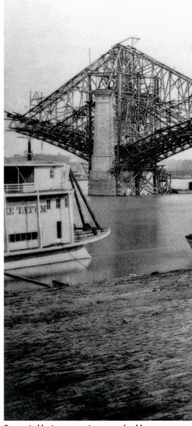
Supported by temporary towers and cables, the steel tubes cantilever outward from the abutment and the west river pier. Robert Benecke, Woodward, History, plate XLIII
