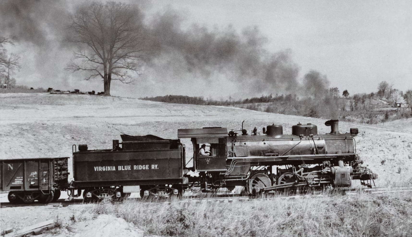
Yes, the camera is level! The 3 percent grade up to Tye River is apparent in this view of 44-inch-drivered No. 7 pulling hard for the Southern interchange. This engine differed from VBR's other Army 0-6-0s in having one large sand dome instead of two smaller ones.
