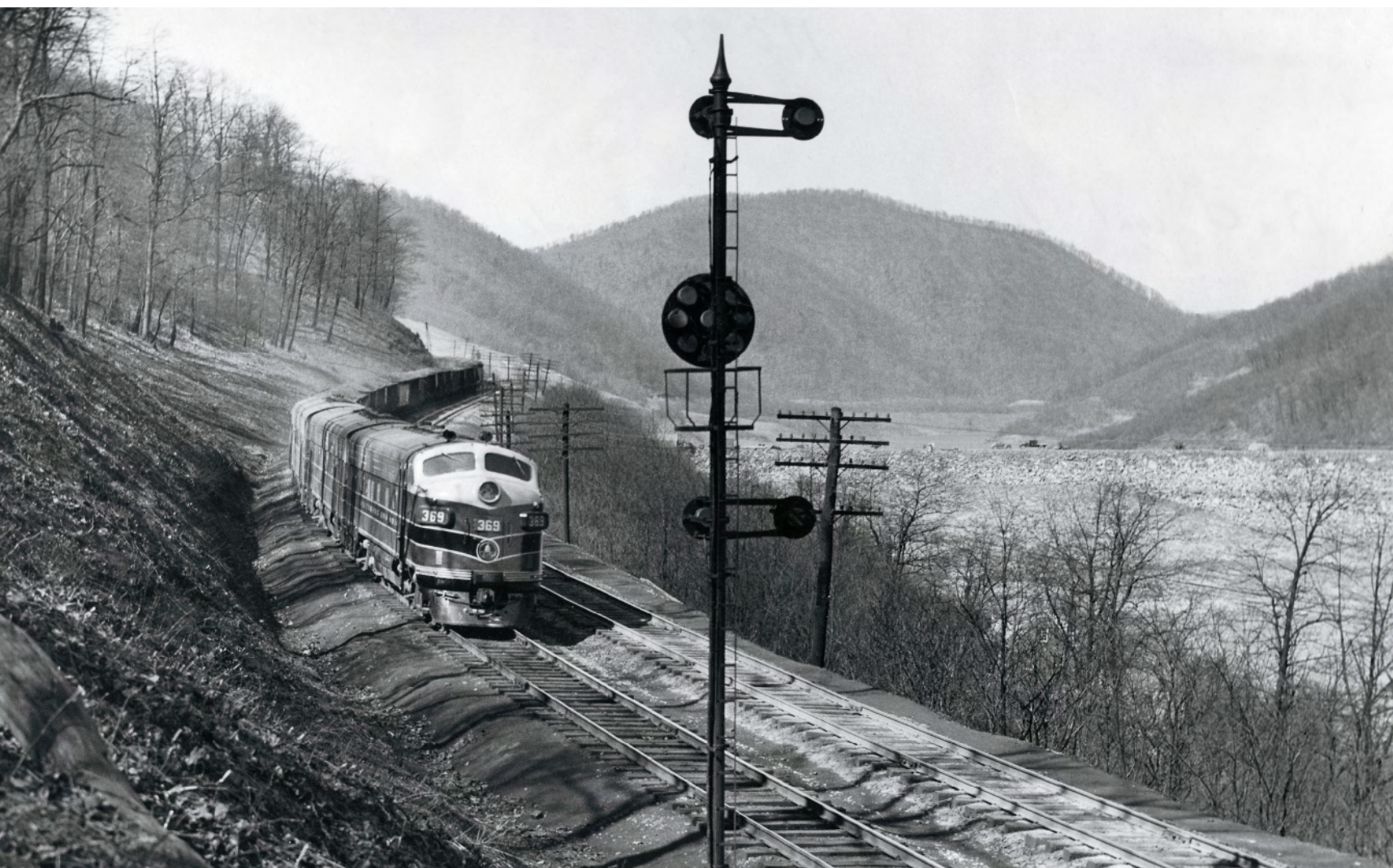
Severe grades made the West End an early candidate for dieselization. In March 1951, dynamic braking on a standard three-unit set of F7's holds back a coal drag dropping down the 2.2 percent of Seventeen Mile Grade at Bond, Md. William P. Price
