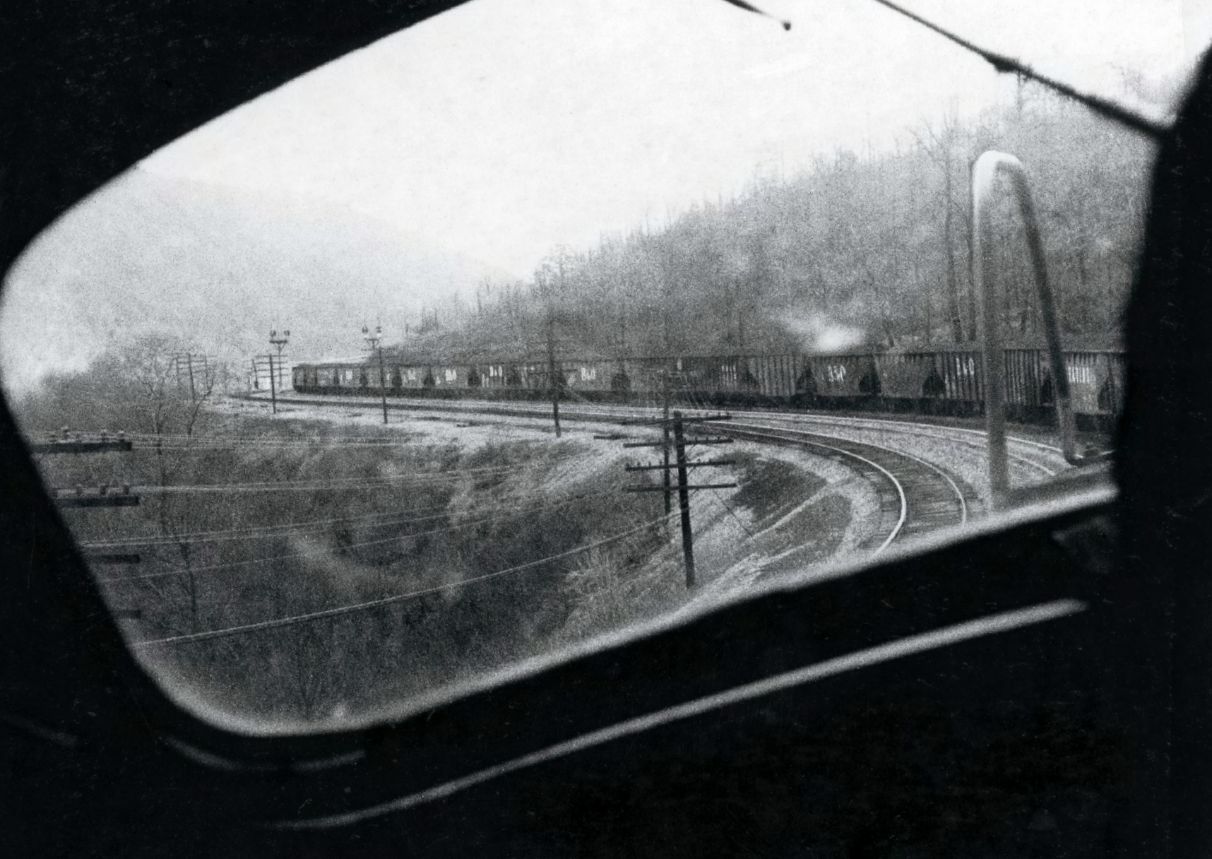
Loaded hopper cars coil through one curve and around another in this late-1959 view from the cab of F7 helper 4493 on Cranberry Grade. Sixty-five cars — 5,900 tons — separate the three units on the head end from the four behind the caboose. Frank E. Shaffer
