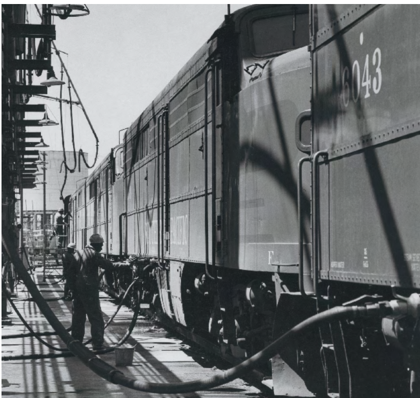
3 Hoses deliver fuel, sand, and steam-generator water to the units. SP had the biggest fleet of PA-family units: 66 PA cabs and PB boosters.
