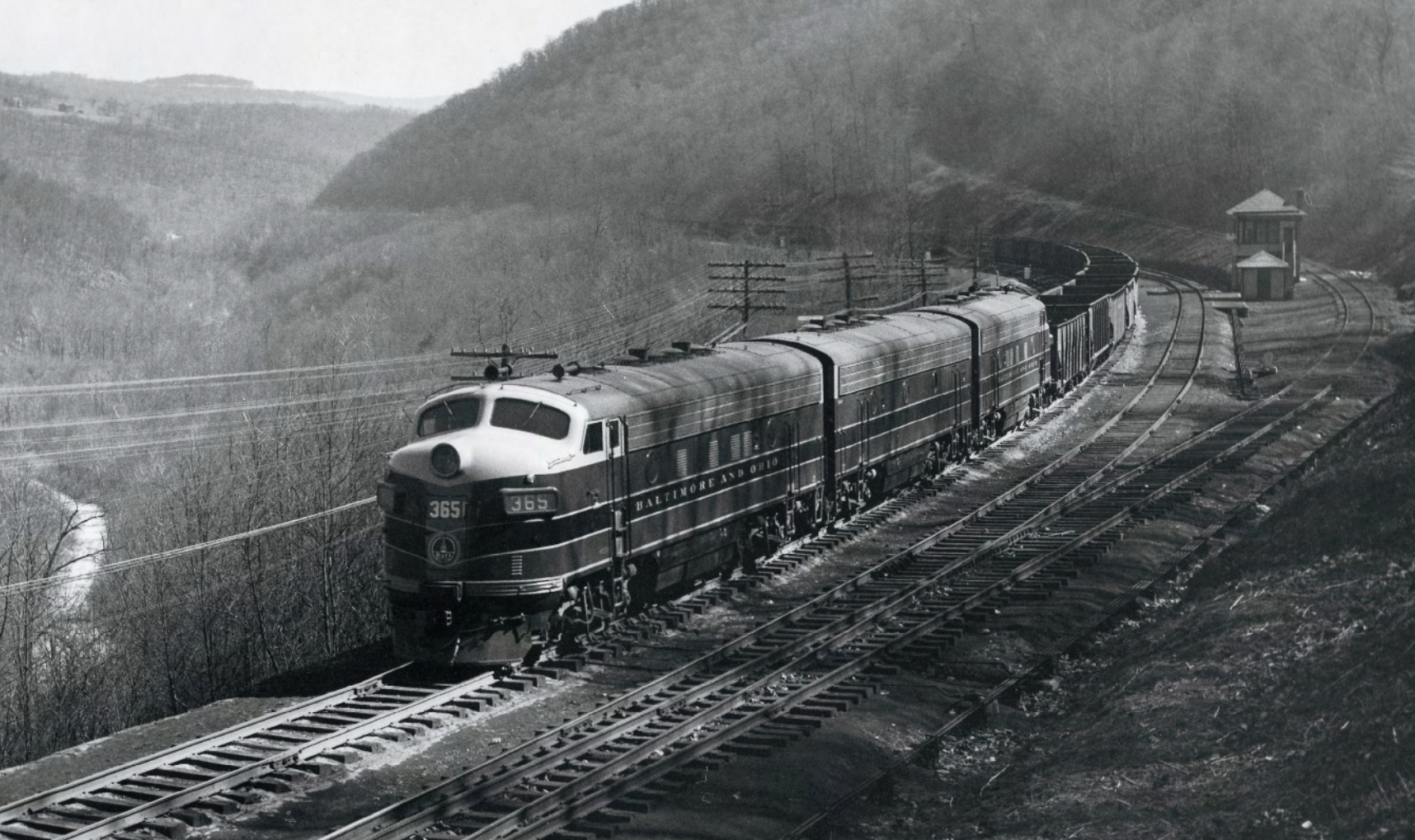
Empty hoppers follow three F7's up Seventeen Mile Grade at Bond Tower in March 1951. Note the safety track curving behind the tower and up the hillside, ready to divert a train running out of control down the hill. William P. Price
