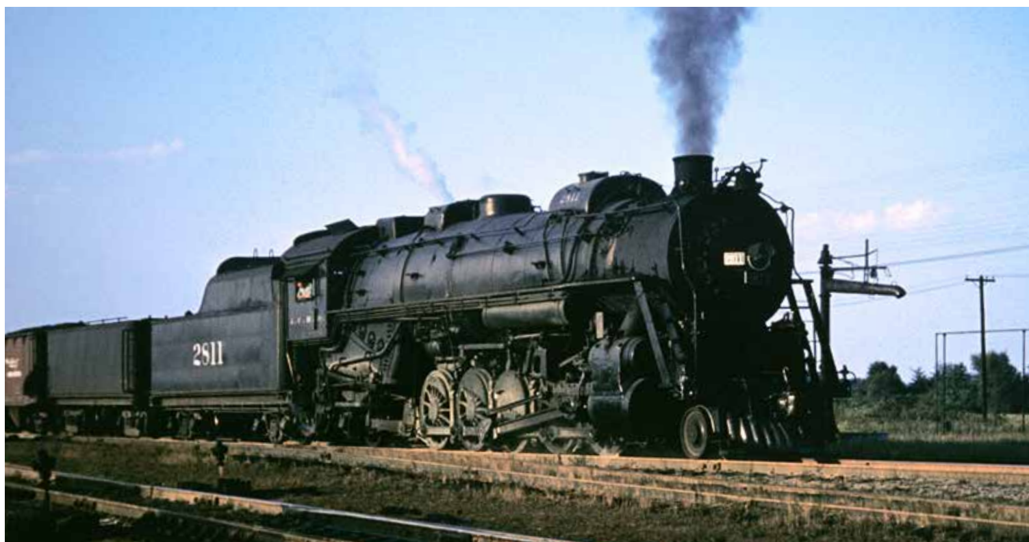
Illinois Central's Paducah (Ky.) Shops kept the road supplied with modern, if no-frills, steam power. IC 2-10-2 No. 2811 (at Carbondale, Ill., in 1957) was built by Lima in 1921; Paducah gave it and 19 sisters new boilers and other improvements in 1944. R. R. Wallin
