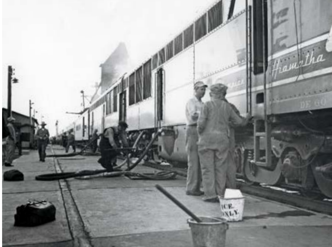
Miles City, Mont., was an important division point, MILW shop town, and train servicing stop, evidenced by the fuel and water hoses connected to the Erie-built diesels on eastbound train 16. Note the OLYMPIAN HIAWATHA lettering on the lead unit. Don E. Wolter
