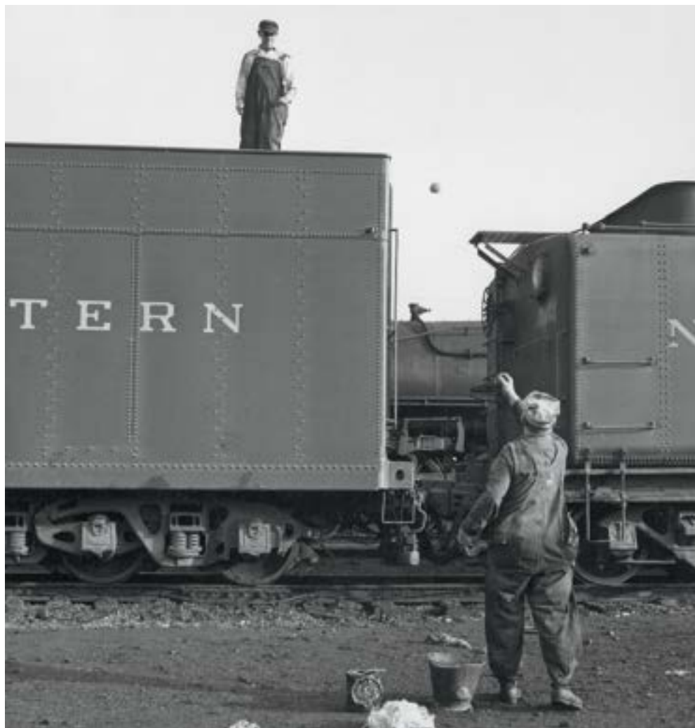
TREATMENT On the N&W at Hagerstown, Md., a crewman tosses balls composed of water-treatment chemicals up to a colleague for him to drop into the tank of a Y6b.
