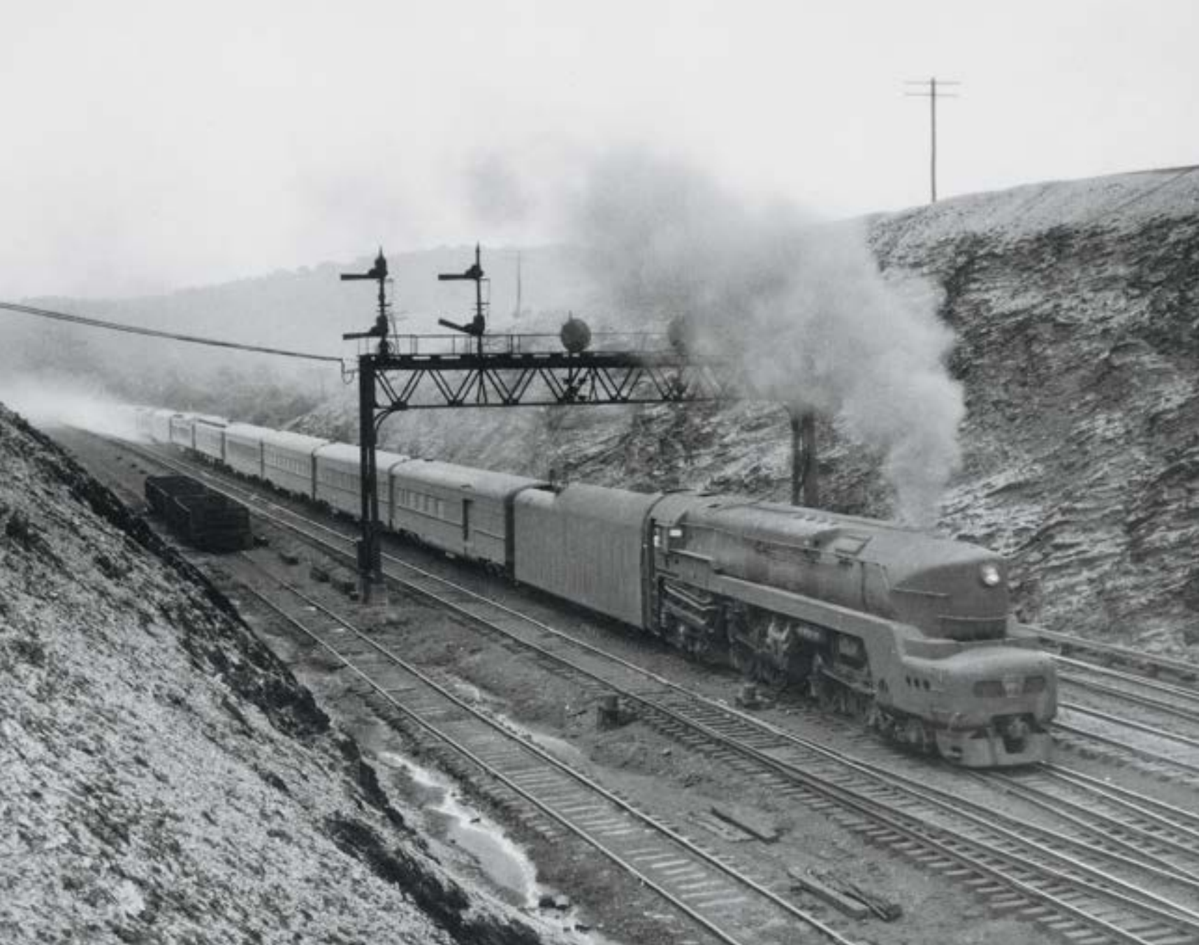
A T1 leaves a cloud of brakeshoe smoke in its wake as it brings a train down off the mountain into Altoona on March 15, 1947. This is the as-built condition of the 50 production T1's, before the addition of steps and number-board/marker-light boxes to the front end.
