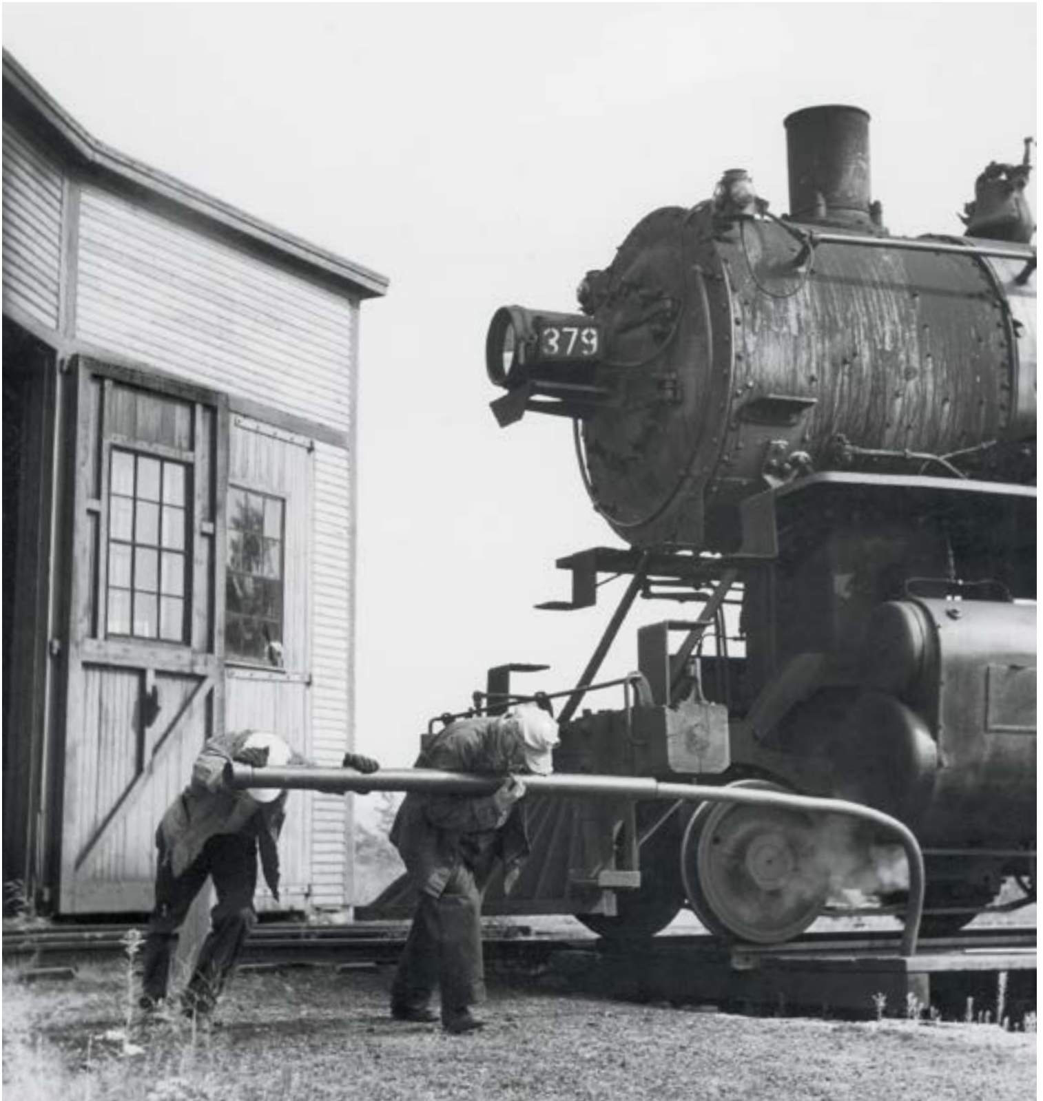
TURNING A TEN-WHEELER: The crew of Maine Central 4-6-0 No. 379 lean into their task on the “armstrong” turntable at Beecher Falls, Vt., in September 1948. The 1907 Baldwin has brought mixed train 378 up from Bartlett and is being readied to return south, with a side trip to Gilman.
