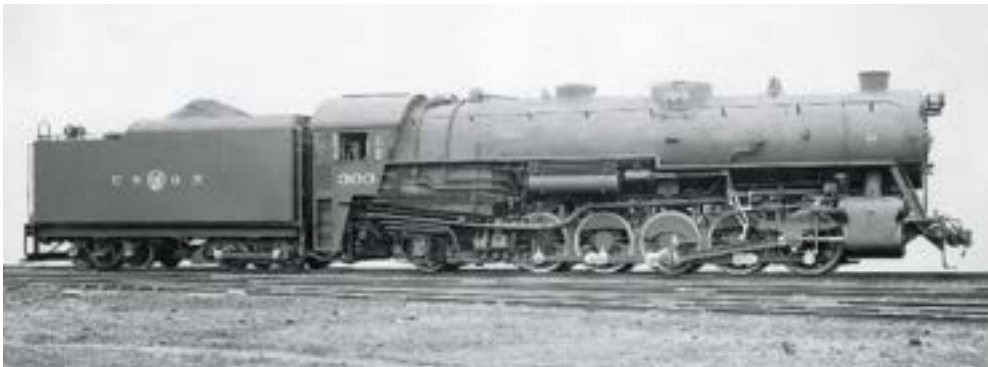
The customary location for the cam boxes was under the right running board, as on 0-10-2 303 (above middle driver), one of five built in 1936 for Pittsburgh's Union Railroad.
