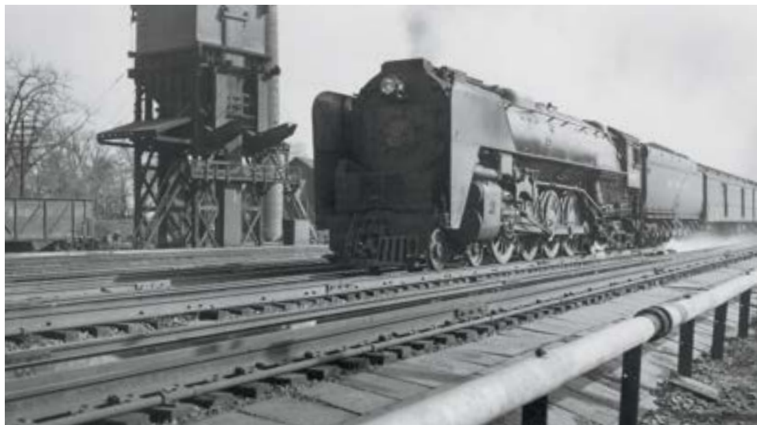
“Down!” A Niagara takes water at the Scotia track pans west of Schenectady. The Central refined scoop and tender-vent designs to enable water-scooping at 80 mph. “Up!”
