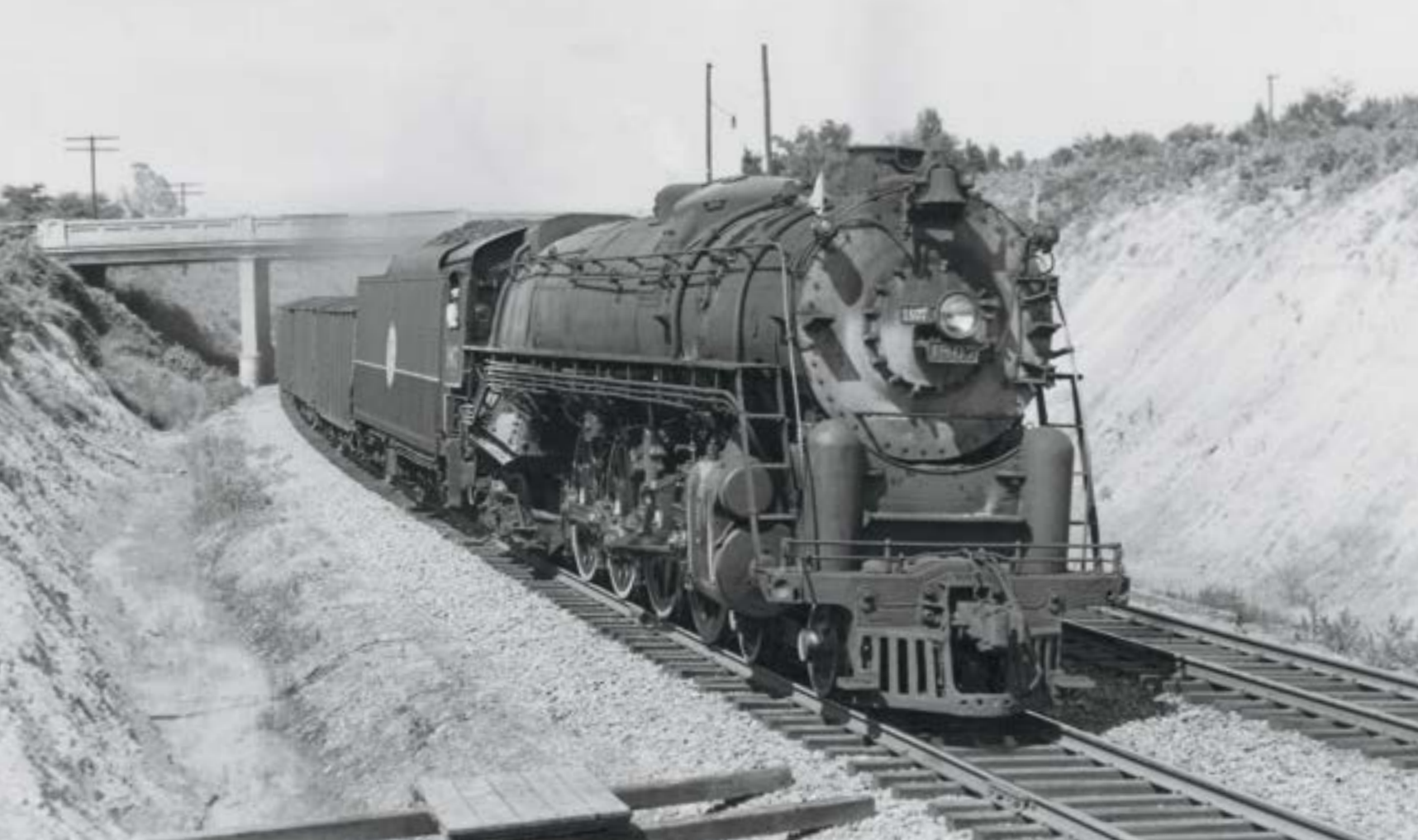
The cam box above the rear driving wheel identifies ACL 4-8-4 1807, heading out of Richmond, Va., with a freight on May 31, 1949, as a Valve Pilot-equipped engine.
