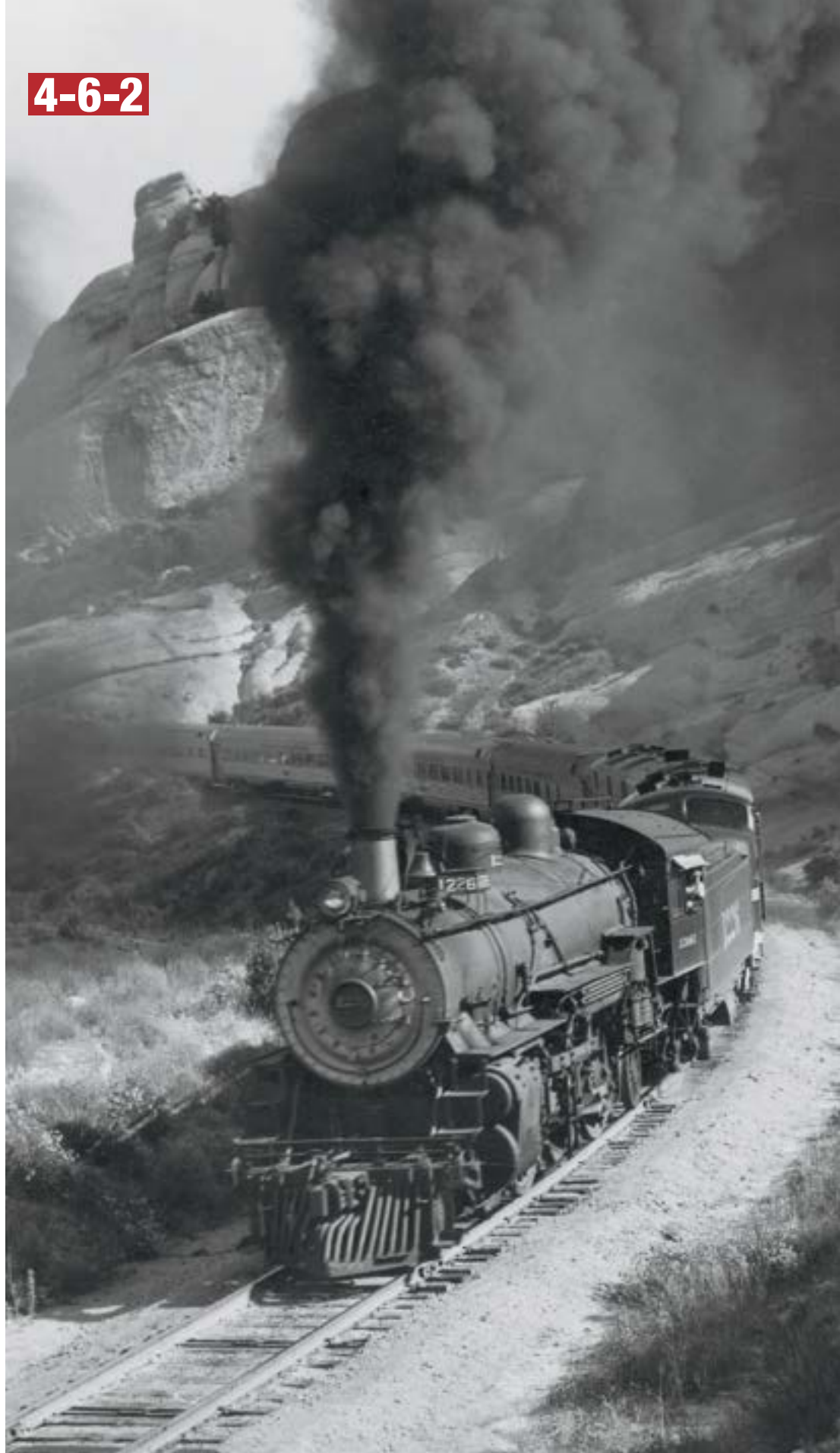
No. 1226 was the first of Santa Fe's second batch of 4-6-2s, built as compounds in 1905. Simplified in 1925, it helps the eastbound El Capitan up Cajon Pass in the early 1940s.
