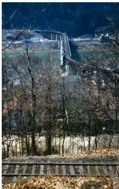
A view from above Foxburg, Pa., shows the two-level (rail on top, road below) ex-P&W bridge over the Allegheny River, with part of the switchback in the foreground.
