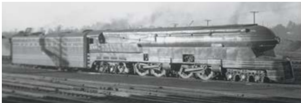
B&O 5600 of 1937 (top, at Washington in 1940) was the first U.S. duplex; it shared a 4-4-4-4 wheel arrangement with the T1, but its rear engine was "backwards." Two years later came PRR's "Big Engine," class S1 No. 6100 (at Fort Wayne in 1941); the colossal 6-4-4-6 was too large for general use, but it sold PRR on the duplex-drive concept.
