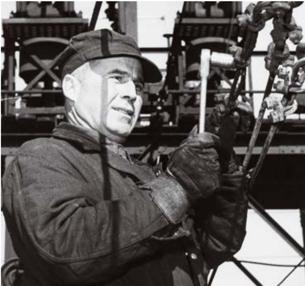
Up on the rooftop platform, a crewman works on a messenger wire, from which the contact wire, or trolley, is suspended by a series of hangers. The messenger wire hangs from two points in the form of a catenary curve, giving the whole overhead system its name.
