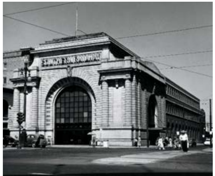
Daniel Burnham designed the Southern's monumental Terminal Station in 1908, just after his Washington Union Station opened. Terminal faced Canal Street at Basin until it was razed in 1956.
