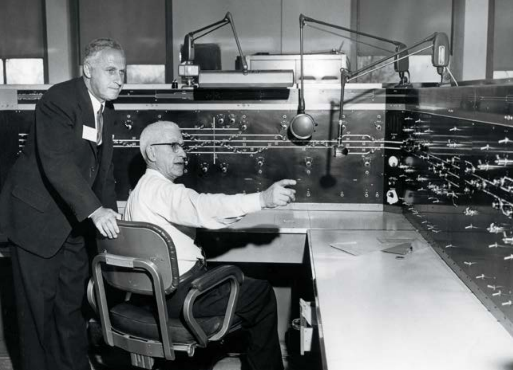
Perlman looks on as a veteran train dispatcher points out the features of a new Centralized Traffic Control console. Rebman Photo Service
