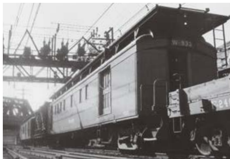
One of the train's old baggage cars is fitted with a rooftop platform on which crews can stand while working on the catenary.
