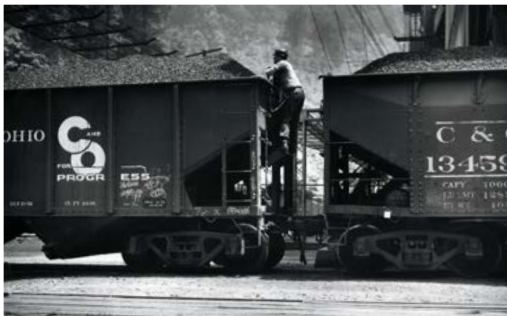
Tethered at the waist to the car for safety, a mine employee rides a string of hoppers that includes Nos. 134594 and 47859 as it coasts from the tippie down to yard.
