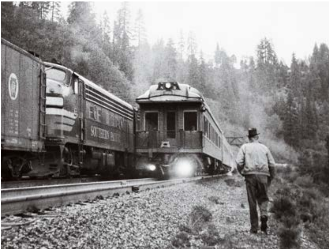
Riding the rear of No. 28, General Manager W. D. Lamprect's business car passes Extra 6311 East's helpers at Midas while the freight's conductor walks forward to inspect his train.
