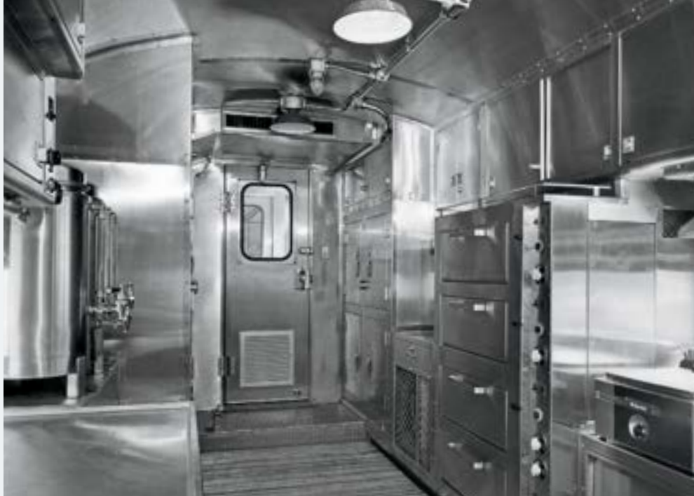
A full-width, 18½-foot kitchen is located in the power car at one end of the train. Light meals and beverages are prepared here and served to passengers at their seats. PRR
