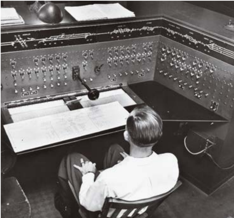
Carl Donald sits before the CTC board from which he directly controls the signals and switches on the line between North Lima and the outskirts of Toledo. Wallace W. Abbey
