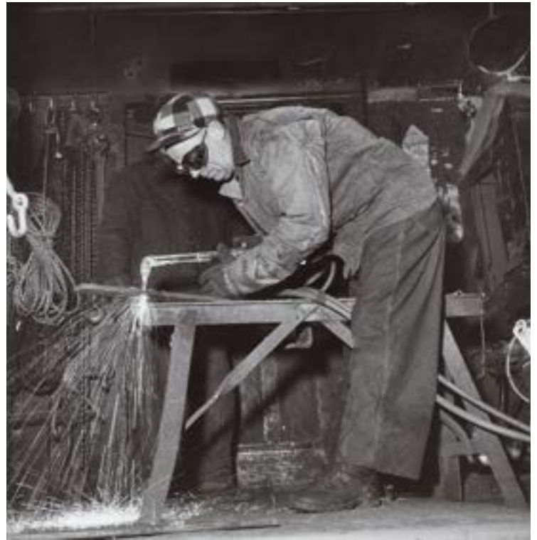
The wire train contains a full workshop. Here, Steve Bettendorf burns a hole in a metal strap used to hang the new transformer.
