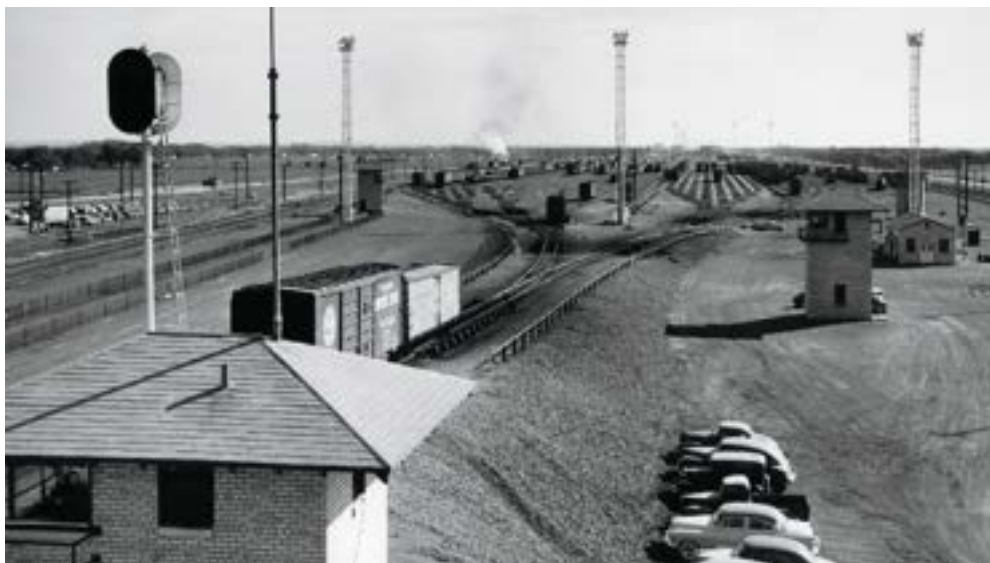
In a view from partway up a light tower, two cars have passed the hump tower and are entering the master retarder. All cars are humped in an eastward direction. Union Pacific
