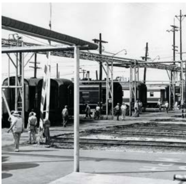
Overhead steam lines frame cars and workers in the coach yard.
