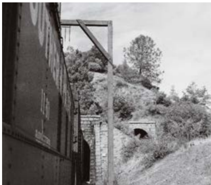
SP caboose 1160 follows its train into Tunnel 23 near Clipper Gap. To the right and slightly higher is Tunnel 22, on the original, steeper alignment used by westbound traffic.
