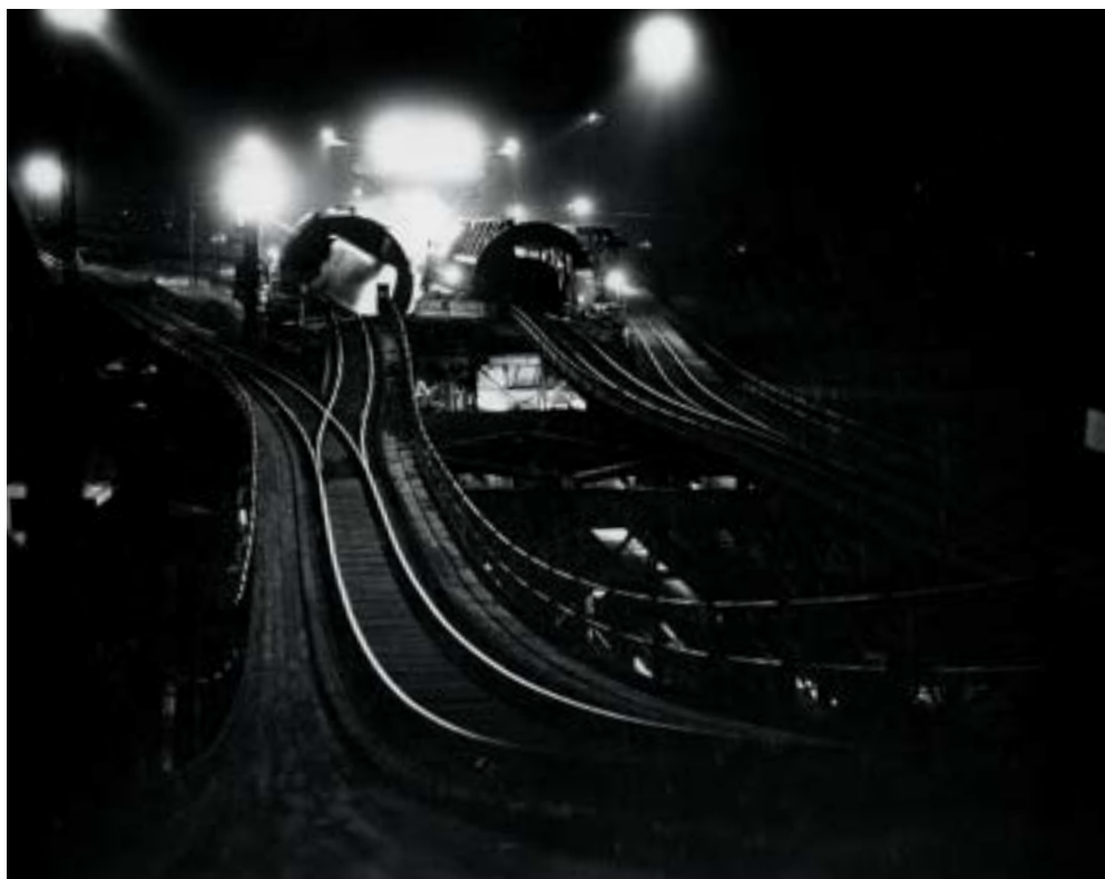
Once unloaded, cars roll out of the dumper toward the camera, up a steep kickback track, and reverse direction down to the empties yard. Later they'll head west for another load.
