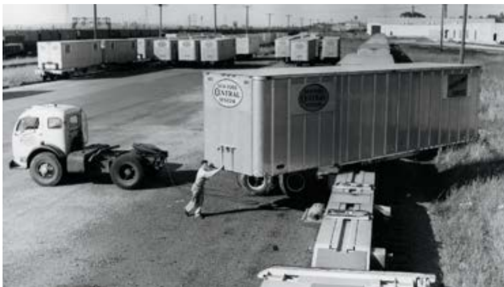
The Flexi-Van system, unveiled in spring 1956, employs truck trailers with detachable wheels that are loaded on special flatcars, saving time, weight, and height. Jim Shaughnessy
