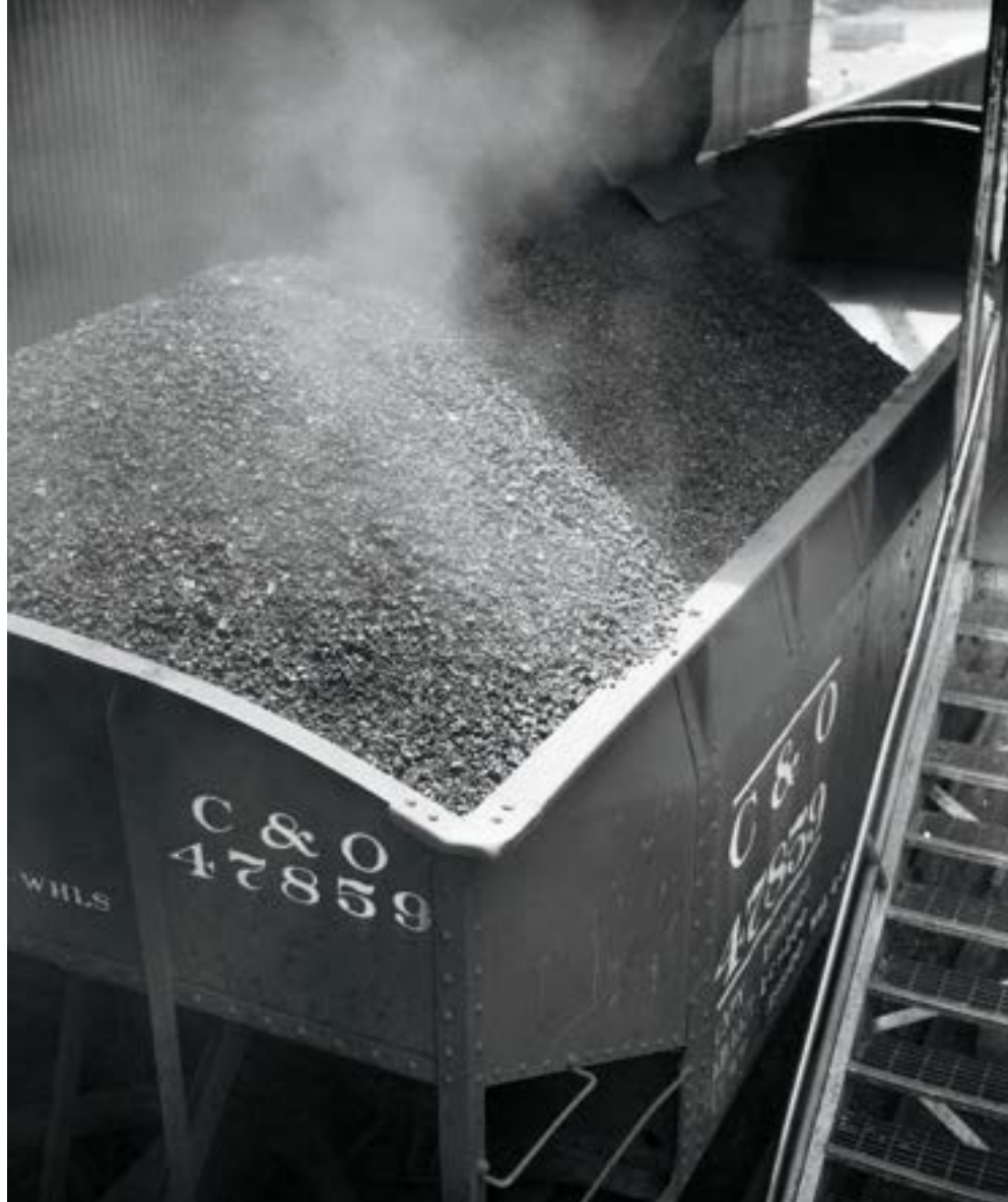
Wharton No. 2’s “inch-and-a-quarter-minus” coke-oven bituminous floods into hopper car 47859, a 1946 product of American Car & Foundry’s Huntington, W.Va., shops.
