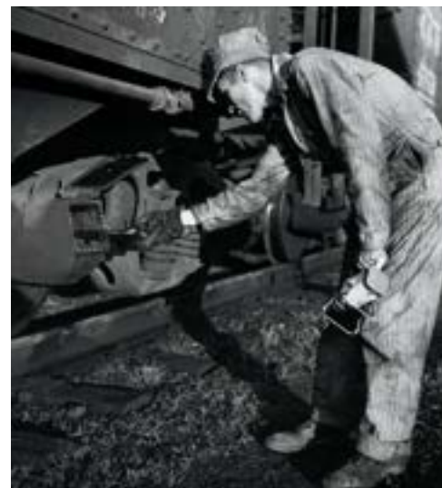
At Danville, a car inspector adjusts the waste inside one of car 134594's journal boxes, possibly preventing a hot box.
