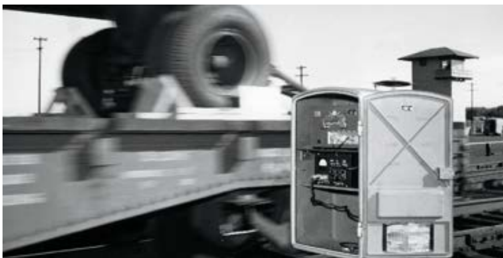
The speed meter, shown with housing cover open, transmits car speed to an "electronic brain" in the tower beyond. This information, along with car weight and other data, determines the force applied by retarders farther into the yard. Union Pacific
