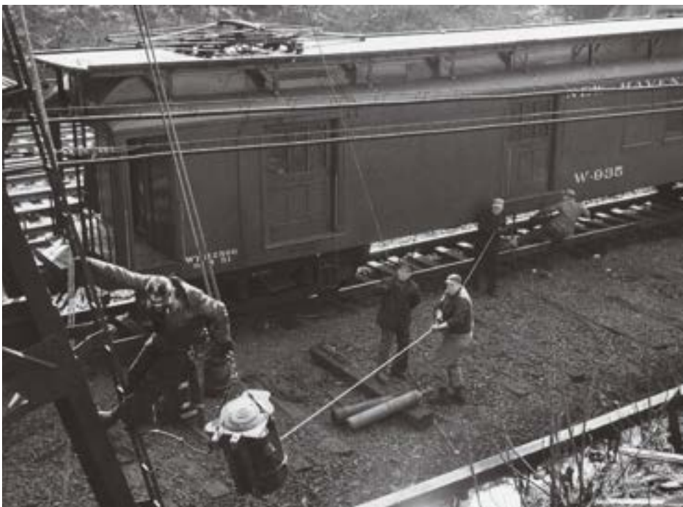
High up on the catenary bridge (upper left), crewmen begin lowering the old transformer, assisted by others on the ground (lower left). With the old unit down, the replacement transformer is hoisted out of one of the cars (above).
