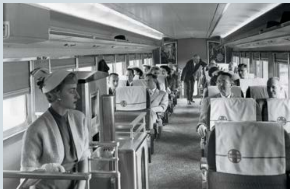
A passenger ascends the central stairway into the upper level of a Hi-Level coach. The low end window beyond the man standing in the aisle shows that this is one of the “step-down” cars with end stairways for access to standard-height equipment. Santa Fe
