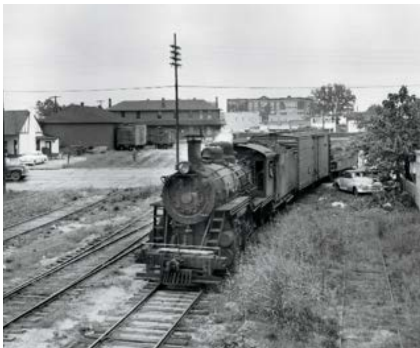
Consolidation 301 switches at Gainesville. The two-story building above its stack is the Midland's headquarters and former depot.
