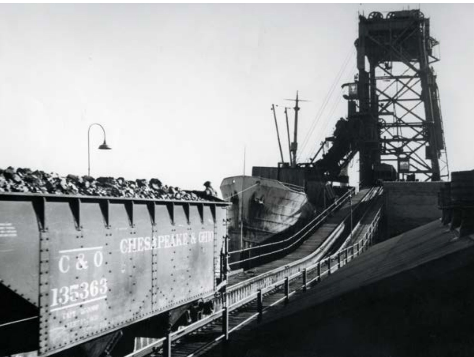
An unseen “iron mule” between the rails propels a coal car, with a brakeman aboard, toward a dumper at Newport News. C&O
