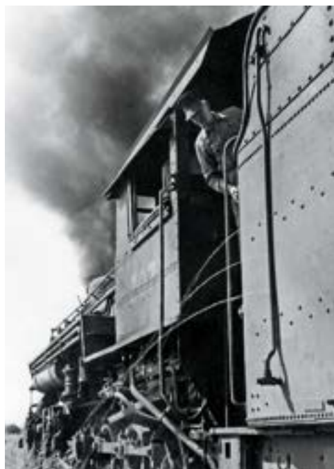
A perforated pipe is used to ascertain the tender's water level. A valve turns off this device when water is not being checked.
