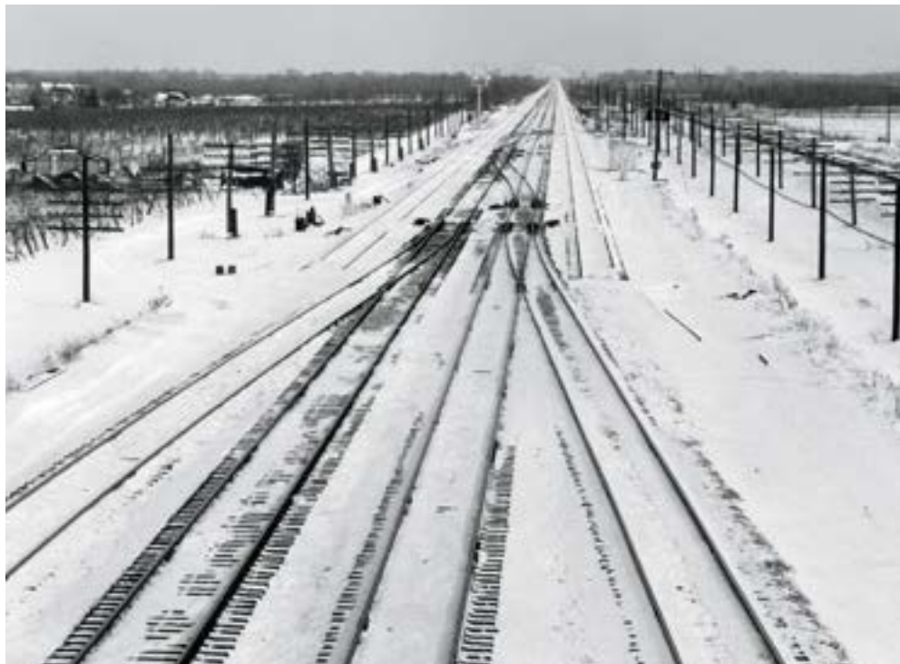
Installation of CTC enabled Central to reduce its Buffalo–Cleveland main line from four tracks to two, with the outer tracks retained in places as sidings. Rebman Photo Service
