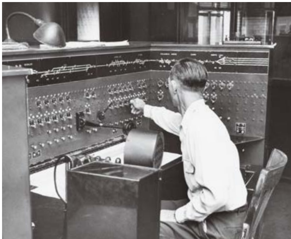
Through the magic of Centralized Traffic Control, dispatcher Donald clears a signal that’s miles away from his office in the second floor of the Deshler tower. Wallace W. Abbey
