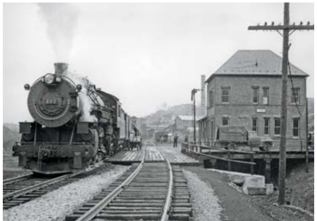
WM Pacific 207 waits as train 1’s baggage-RPO is loaded at Thomas on April 29, 1951. From here, at an elevation of 3,000 feet, it’s downhill to Black Fork Gorge. K. F. Merlin
