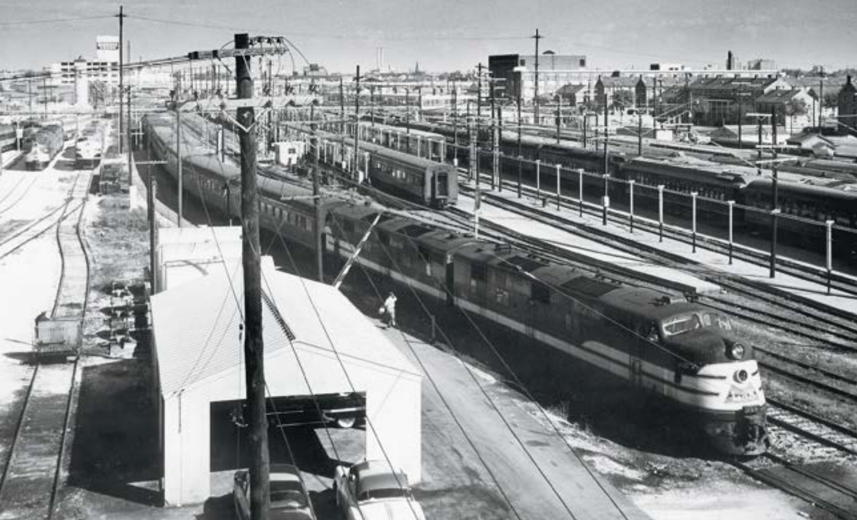
Having turned on the wye, L&N's Humming Bird passes between the engine terminal and coach yard as it backs toward the station.
