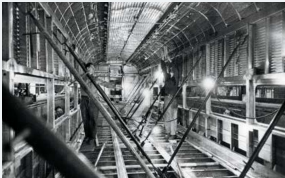
While conventional cars rely on a center sill and heavy underframe for strength, the Tubular concept incorporates the sides and roof into the overall structure. Budd Co.
