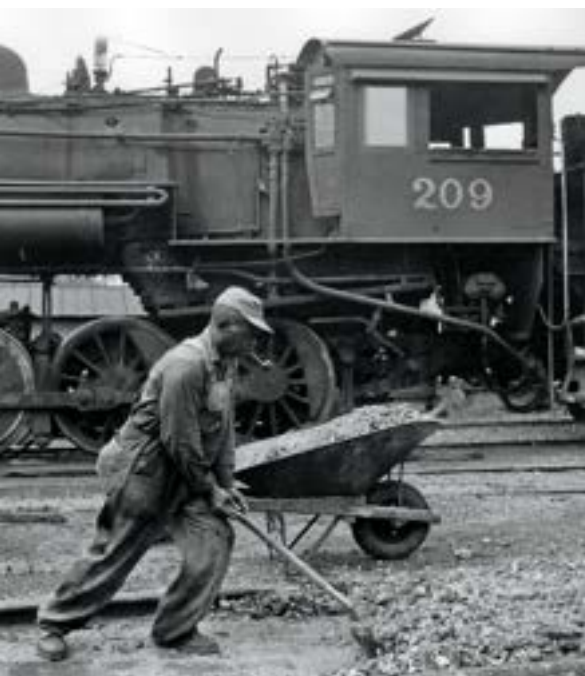
Ash disposal, GM-style: cinders are dropped between the rails, shoveled into a wheelbarrow, and dumped on a flatcar.
