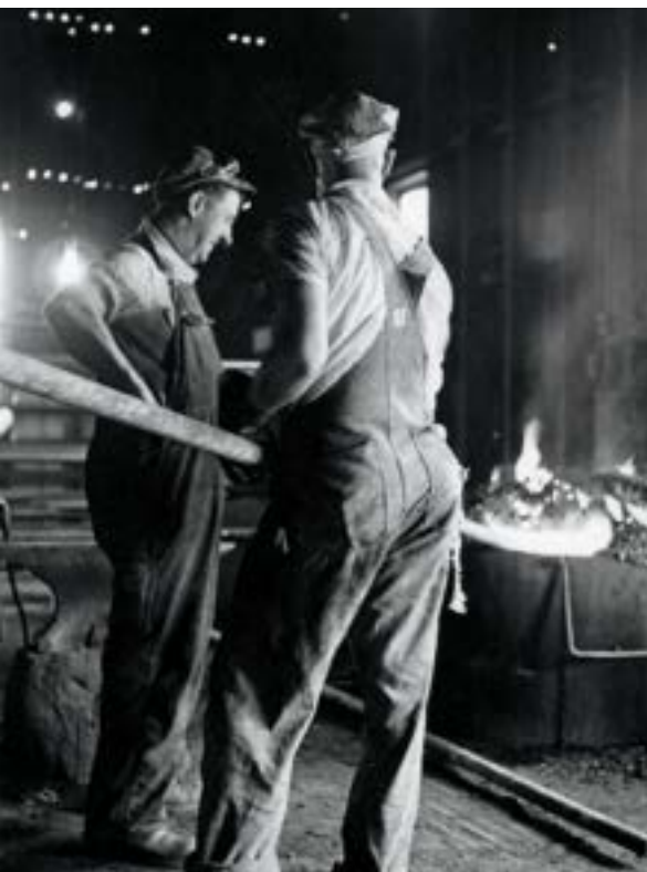
This April 1957 scene of two Midland men annealing the ends of a flue for Decapod 208 would be familiar to shopmen of 100 years earlier. The short line used to send its flues to the Seaboard shops for machining, but now must do the work itself, by hand, after the disestablishment of steam repair facilities on the big road.
