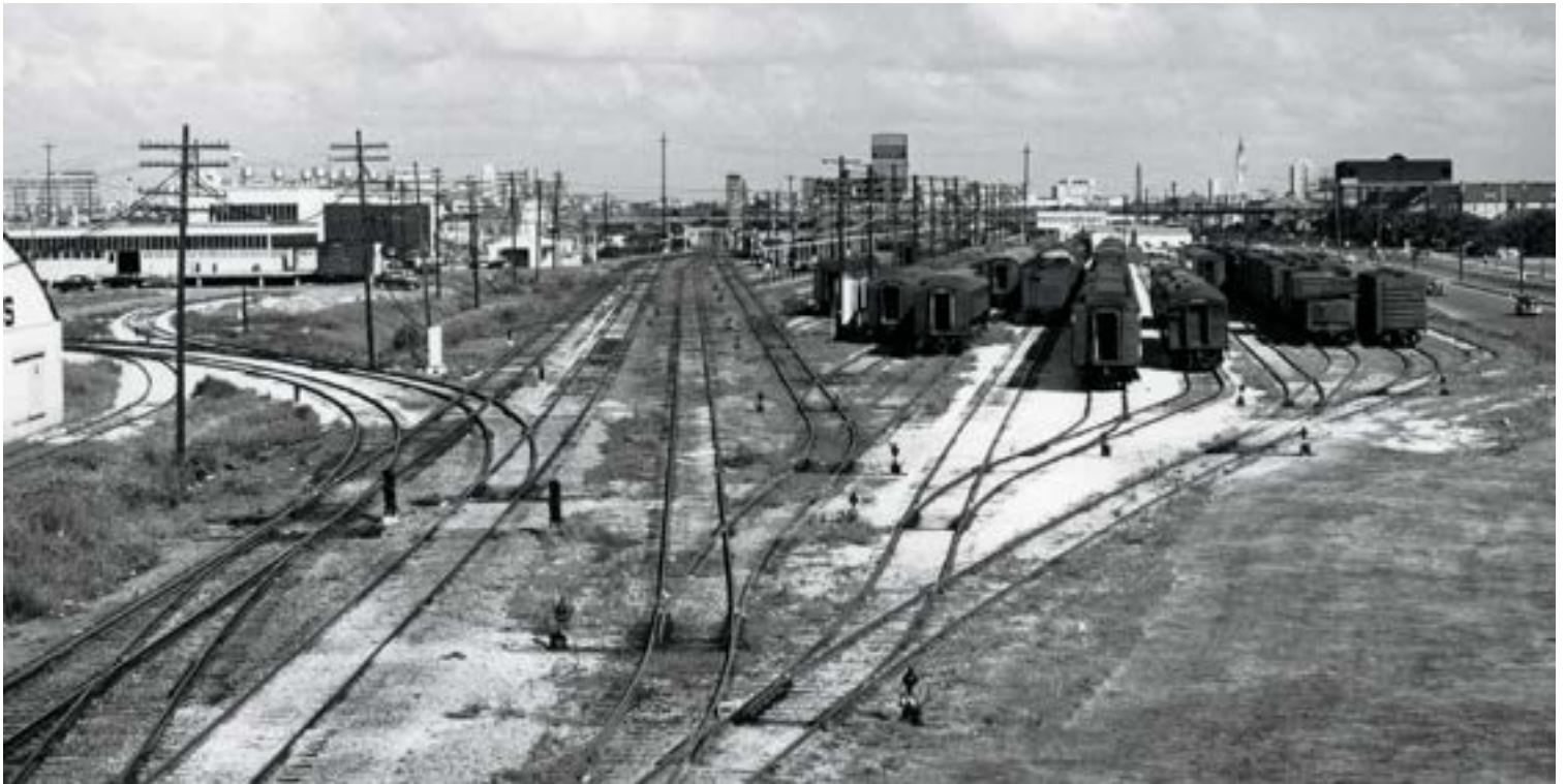
The South Wye switches (controlled by Clara Street tower) and the coach yard dominate a view south from the Broad Street overpass.
