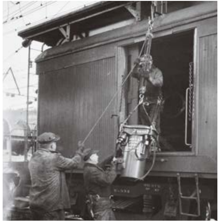
High up on the catenary bridge (upper left), crewmen begin lowering the old transformer, assisted by others on the ground (lower left). With the old unit down, the replacement transformer is hoisted out of one of the cars (above).
