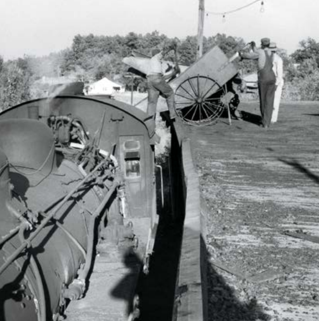
All locomotives take coal at Belmont — because that's where the Midland's only coaling station is located. Men tip and shovel a cart of fuel from a platform into No. 207's tender.
