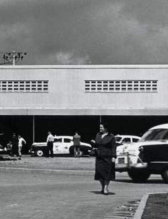
Taxis and private autos wait at the cab stand on the east side of the terminal. A limestone facade visually unifies the main building (left) with the baggage room. Between the two, beyond the three people walking, a heavyweight Pullman is visible.
