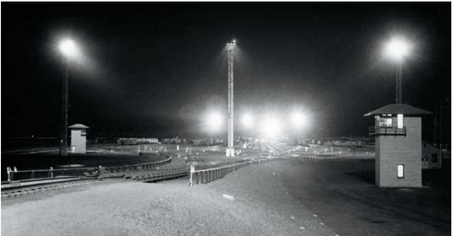
North Platte by night: An eastward view from the hump into the 42-track yard shows Towers A (right) and B. These structures, along with Tower C (hidden by Tower A) control retarders that slow the cars and switches that route them to the proper track. Wallace W. Abbey
