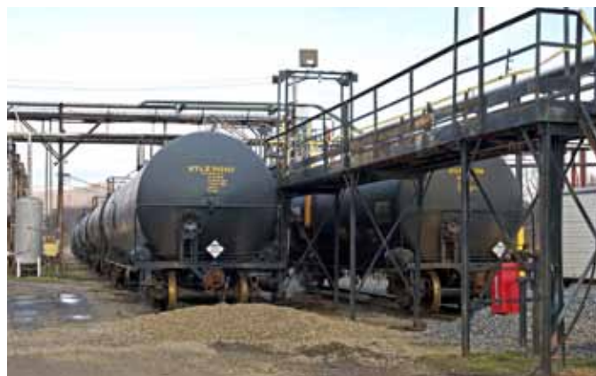
Overhead piping transfers raw materials and finished products between the plant and these tank cars. The overhead rack is similar to Walthers' HO Cornerstone kit.
