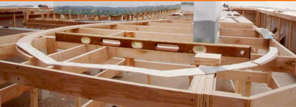
For the WP First Subdivision, Tommy used 3/4" birch plywood in 8-foot super dominoes for the benchwork. This photo shows the benchwork in progress.
