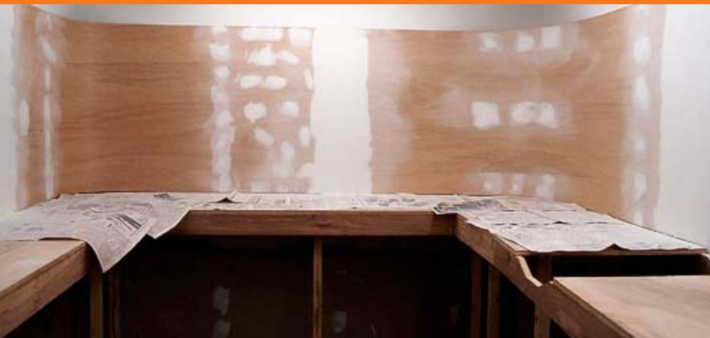
On most of the layout, Tommy used wallboard for the backdrop. However, where coved corners were required, he used 1/16" door-skin plywood.
