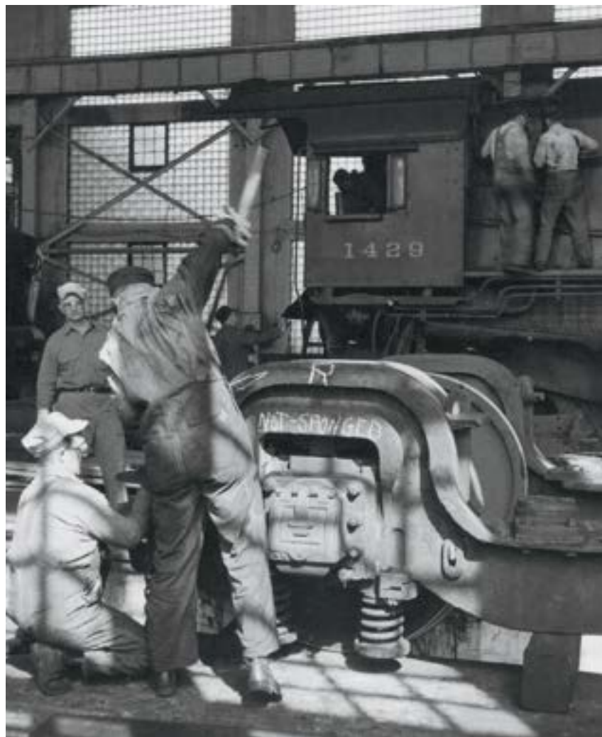
Ready for re-wheeling, L1 1429 waits in the wings while workers prepare her trailing truck.
