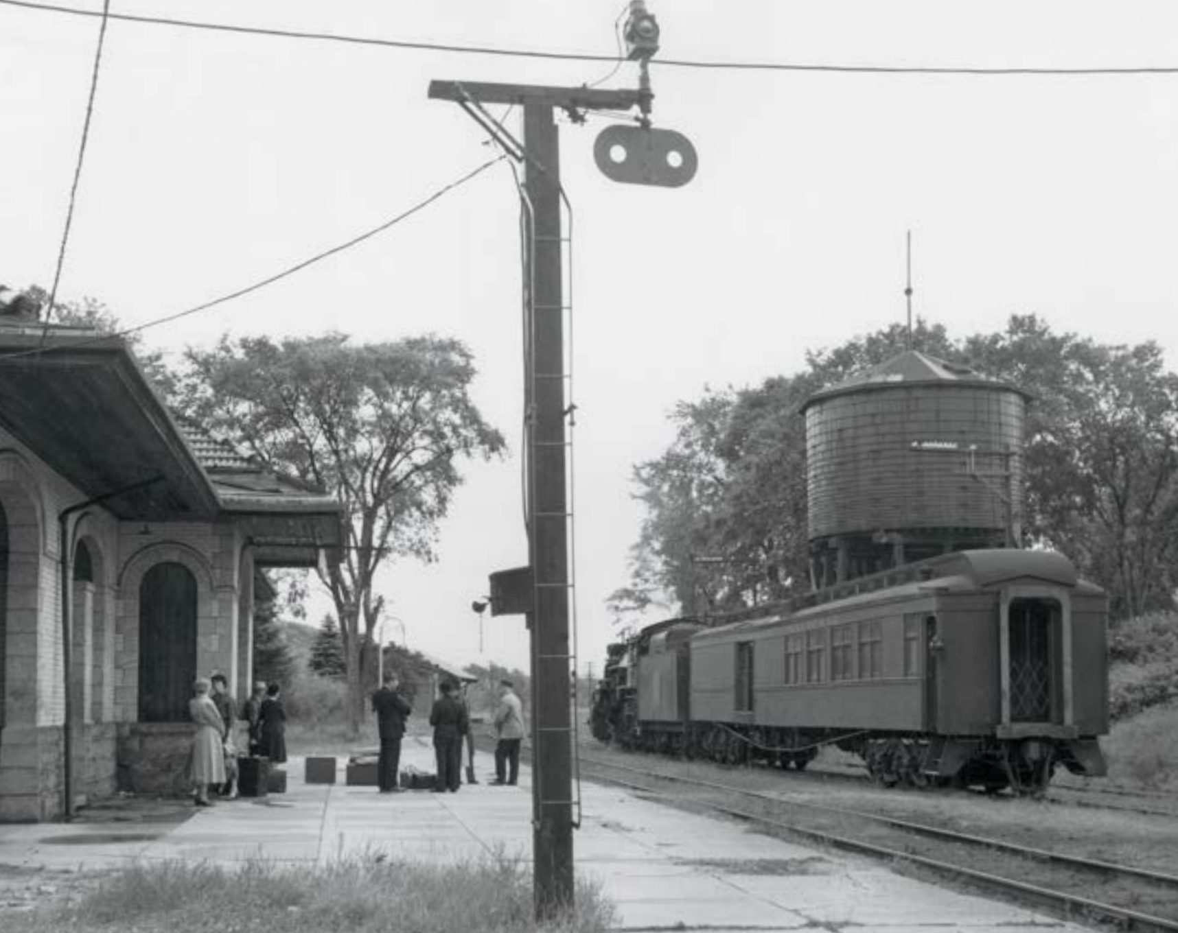
Connection at Danville Junction, Me., — like the Lark in San Jose ...
