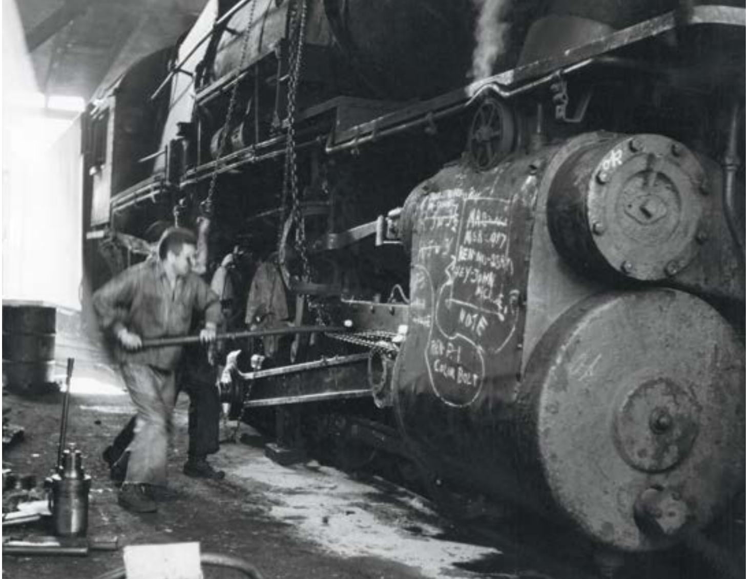
Shop men struggle with block and tackle to remove an I1's main rod.
