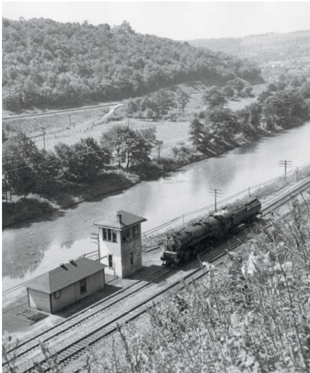
Helper crew confers with GA Tower operator.
