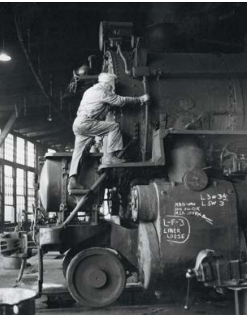
Doctor's orders chalked on her steam chest, I1sa 2-10-0 No. 4230 undergoes running repairs in the roundhouse.
