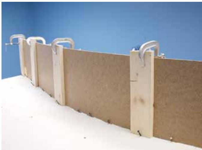
C-clamps at the top of the backdrop and drywall screws at the bottom force the back-to-back pieces (rough side to rough side) of tempered hardboard together until the carpenter's glue dries.
