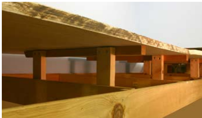
Fig. 5. Check for obstructions. Risers allow adjusting the level or grade of baseboards, but may interfere with turnout motors or other devices. Paul leaves all the screws exposed in his risers and joists so any of them can be moved.
