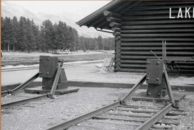
Heavy-duty bumper posts are typically found on heavily used spurs or where buildings are located directly behind the end of the track. Glenn A. Wagner photo
