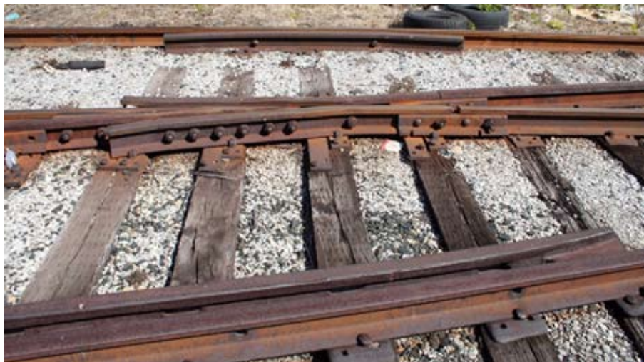
Here's the kind bolt detail along the frog wing rails that can be modeled with the add-on parts included with the Micro-Engineering turnout. To the right of the frog are the joint bars connecting the frog to the closure rails.
