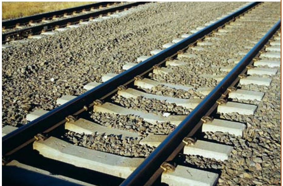
Concrete ties, such as these on the Union Pacific near Lewellen, Neb., can be found on many main lines throughout the country. Concrete ties tend to be wider than wood ties, and more widely spaced. The contour drops in the middle, and ballast often covers the middle of the ties. Jeff Wilson photo
