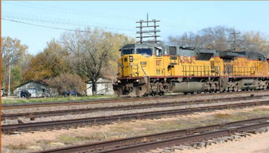
The two mainline tracks on this Union Pacific line have a high ballast profile with welded rail. The next nearest track is a passing siding, which also has welded rail but a noticeably lower ballast profile. The two nearest tracks are spurs to a grain elevator. They are at ground level, have jointed rail, and have little to no ballast. Jeff Wilson photo
