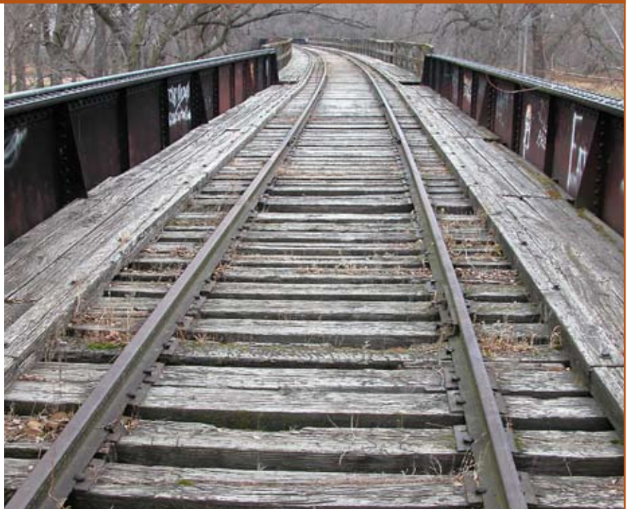
On an open (or unballasted) bridge deck, ties are spaced much closer together than in standard track. Jeff Wilson photo
