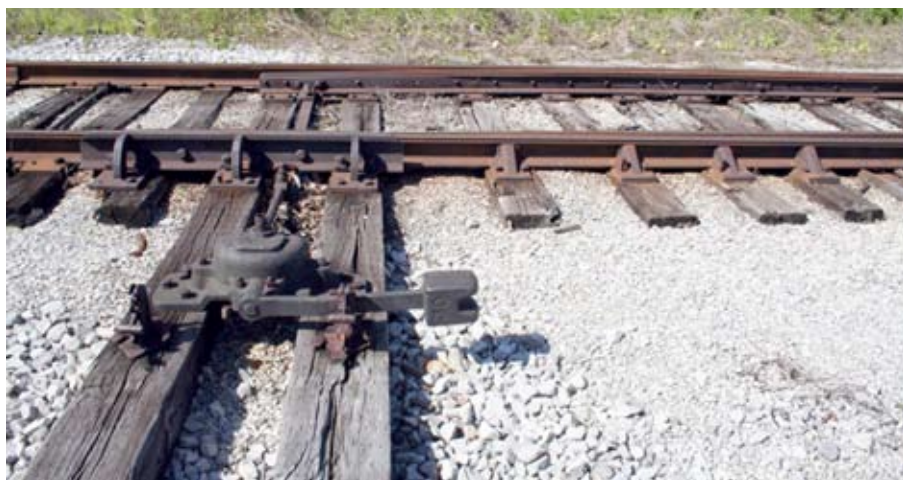
The headblocks, the extended ties at the point end of the turnout, serve as a rigid mounting for the switch stand. Other details here include four rail anchors along the stock rail to the right, and a switch point protector or guard. This raised, outside guard rail deflects wheel flanges away from the tip of the point to reduce point wear and prevent flanges from picking the point.
