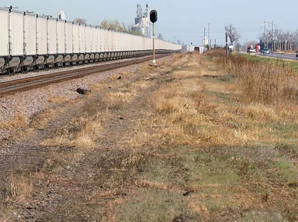
This well-maintained double-track Union Pacific main line in Nebraska has welded rail on both lines, anchors at every tie, and a tall ballast profile. The line sees dozens of trains each way every day, including many heavy unit coal trains. Jeff Wilson photo
