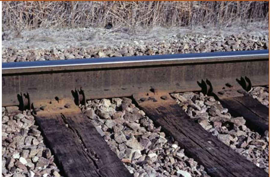
This mainline track has wide tie plates spiked to the tie separately from the rail spikes, with rail anchors installed on both sides of every other tie to prevent the rail from creeping. Gordon Odegard photo
