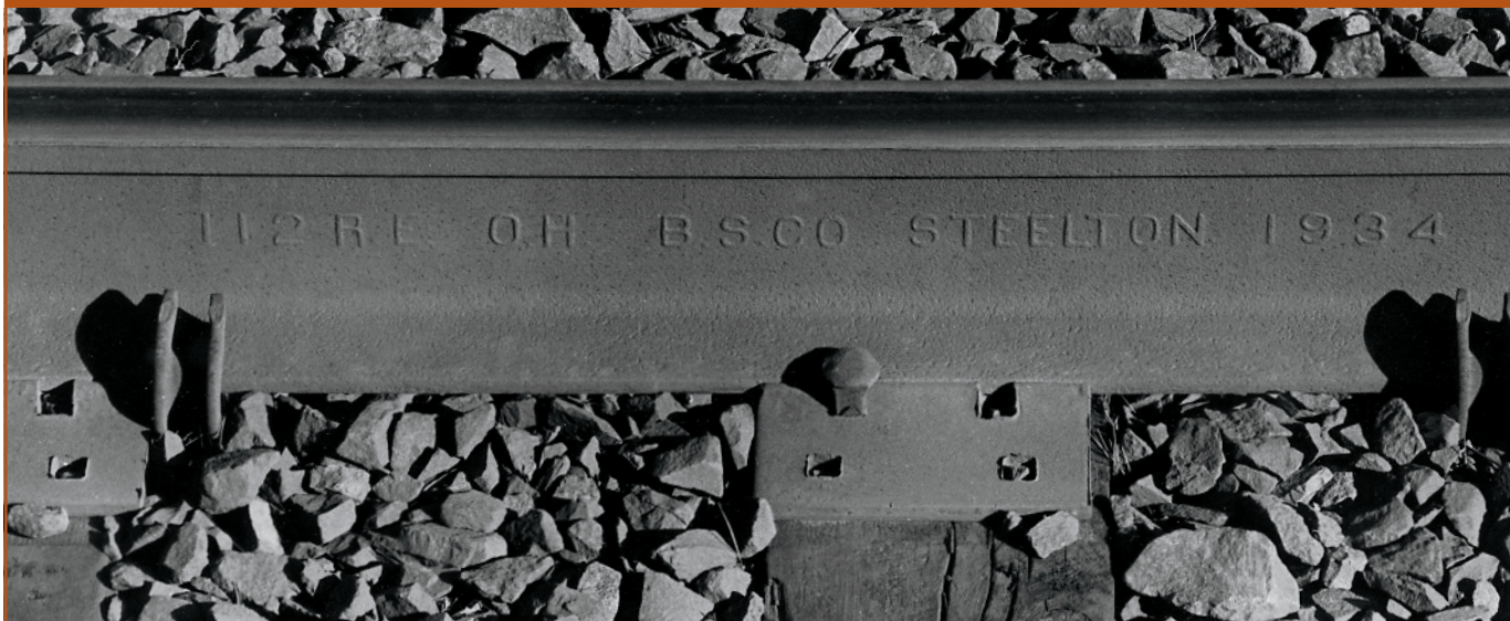
Rail is labeled with the maker and weight. This 112-pound rail was rolled at Bethlehem Steel's Steelton, Pa., plant in 1934. It is in service here on Conrail in 1978. Tom Nelligan photo
