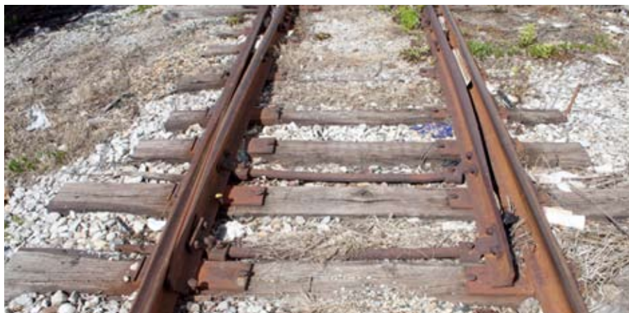
The moving parts of the turnout, the points, are called the switch. Here you can see the two switch rods that connect the points so they move as a unit. The left point of this switch is spiked and the switch stand has been removed, so the diverging leg of this turnout is apparently out of service.
