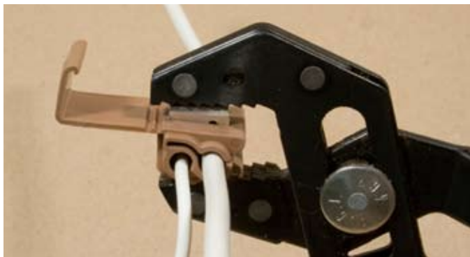
Fig. 6 Squeezing the knife. Andy uses Robo-Grip cam-action pliers to press the connector's knife flush with the body of the connector. The knife cuts through the insulation and into the metal conductors, bridging the two wires together.
