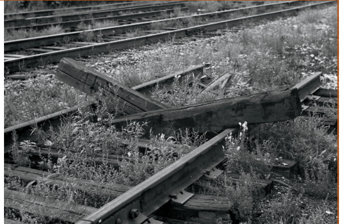
The ultimate in cheap track bumpers is a pair of ties buried in the roadbed. A pile of dirt or ballast could serve the same purpose. Harold Russell photo
