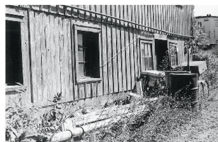
Along the lower level in back, some battens are conspicuous by their absence, worth duplicating on a model. The signal department used the area for storing signal masts and other hardware.
