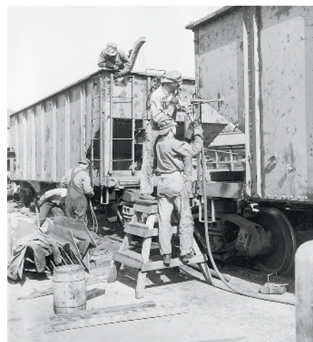
Air-powered tools are common equipment at RIP tracks, as are a variety of ladders and access stands. Trains photo by W.A. Akin Jr.
