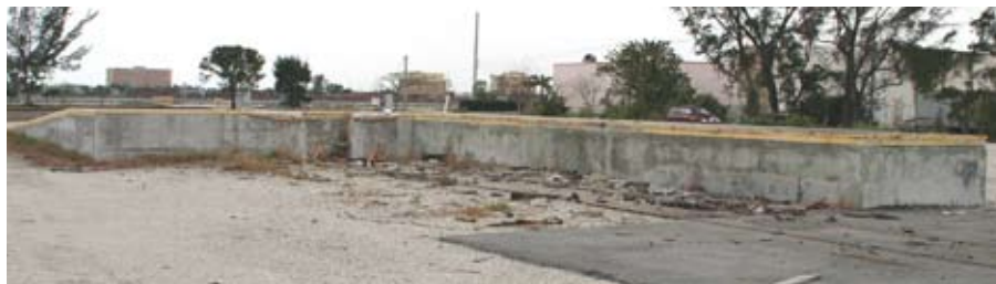
Fig. 5 Dock shape. Some ramps include a dock extension alongside the track so loads may be shifted on or off cars from the side.
