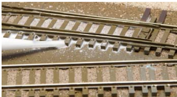
Fig. 5 Stuck no more. Are you tired of having ballast glue sticking switch points to the ties? Try applying the glue from the side. Cody saturated the ballast until the Scenic Cement was visible between the granules.
