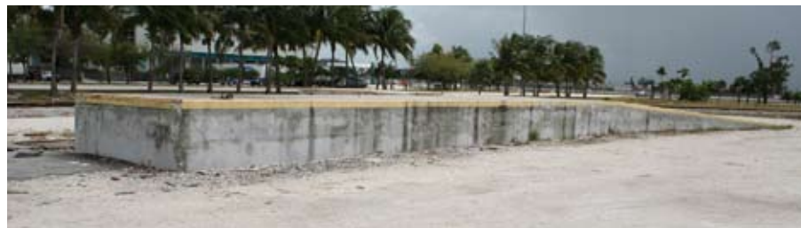
Fig. 4 Form marks. The sides of concrete ramps are typically covered with a variety of marks left by the wooden forms used in pouring the concrete.
