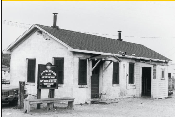
The four main walls of the westbound yard office are made of concrete blocks. Visible in this 1971 photo, a wooden vestibule was added to the main entrance during the steam era.
