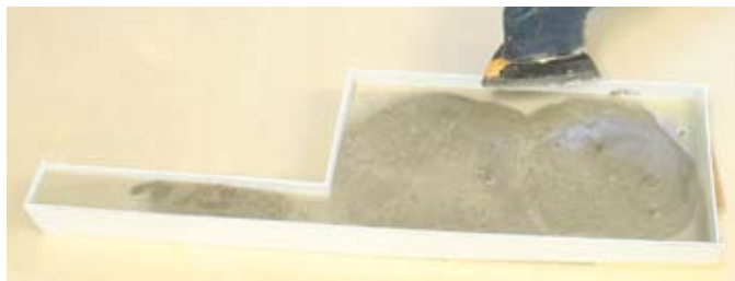
Fig. 7 Vibrating the form. Lance held a small power sander against the edge of the form so its vibration would free air bubbles trapped in the poured wet cement.
