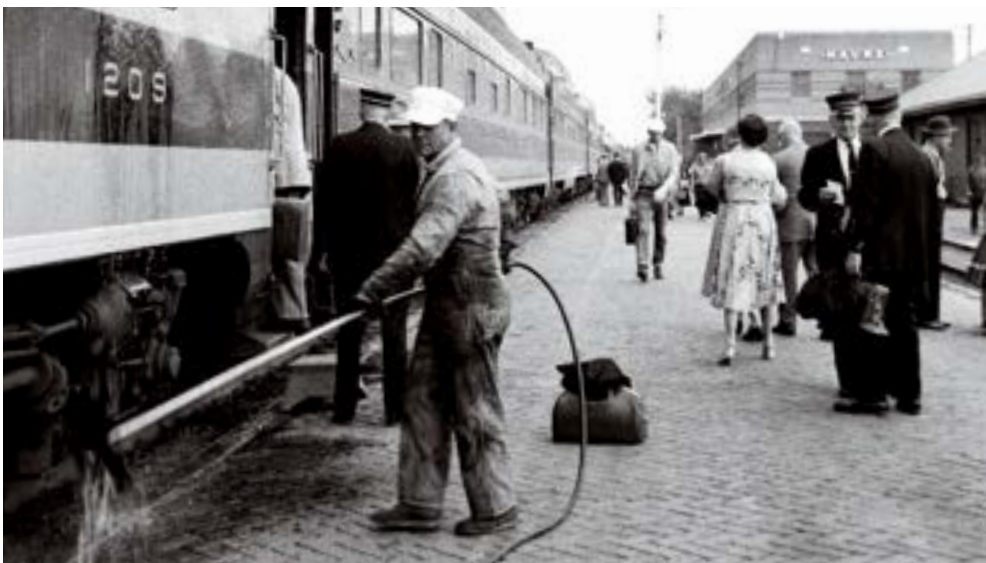
During the 11-minute stop at the division point of Havre, Mont., the Builder's train and engine crews are changed and the locomotives and cars are fueled and watered.
