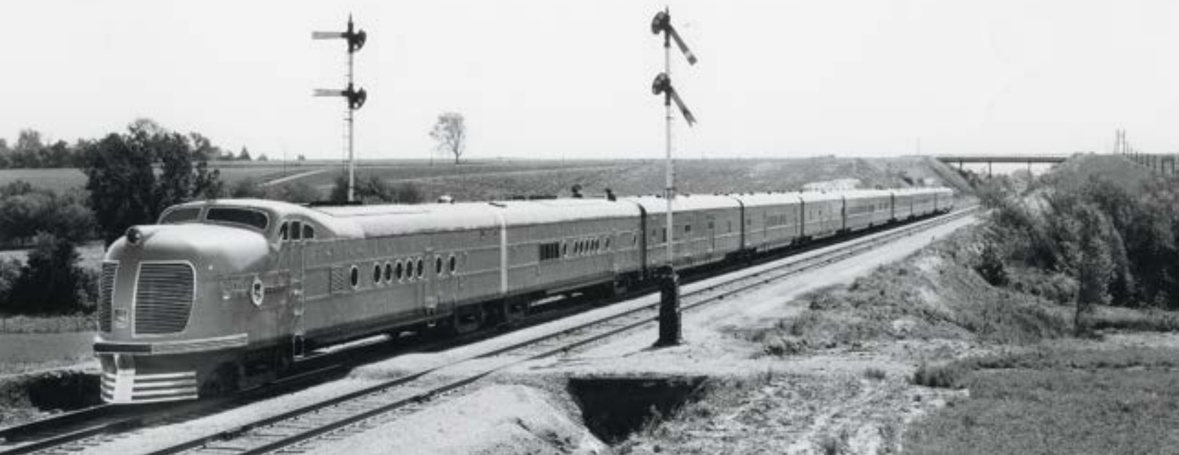
Brand-new in mid-1936, one of the two City of Denver trains poses on the Lane Cutoff west of Omaha, a favorite spot for UP publicity photos. The portholed cab and booster units rode on two trucks each, but were connected by a span bolster, not couplers.
