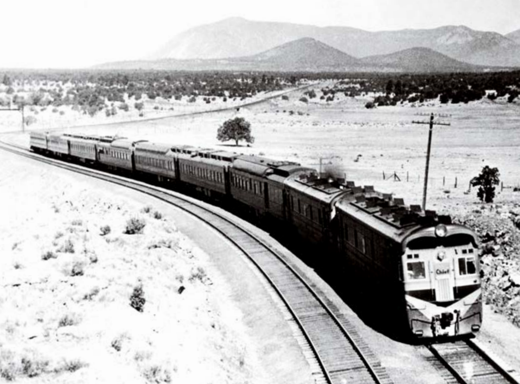
Two-unit box-cab diesel No. 1 is eastbound with the first, heavyweight iteration of the Super Chief about 15 miles east of Flagstaff, Ariz., in mid-1936. The B-B, twin-engine, 1,800 h.p. units were based on Electro-Motive demonstrators 511-512 and B&O 50.
