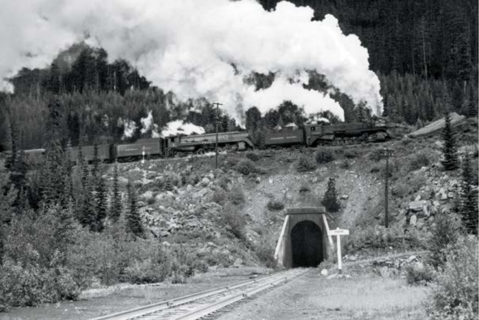
A 2-10-2 helper and 2-10-4 road engine thunder up Kicking Horse Pass with the eastbound Dominion in June 1949. Minutes earlier, the train disappeared into the portal below the engines to negotiate Spiral Tunnel No. 2, the lower of the two curved bores.
