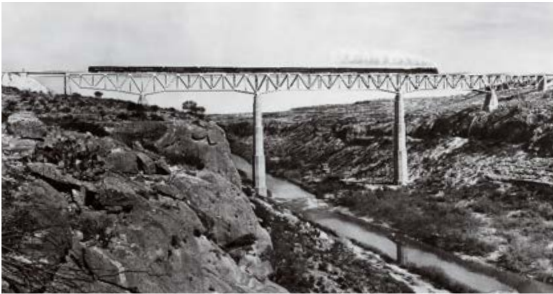
Although much shorter than the Huey Long Bridge, SP's crossing of the Pecos River, 65 miles west of Del Rio, Texas, stands more than twice as high: 362 feet above the river. It opened in 1944.
