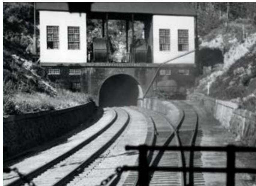
The mountain obs cars afford a fine view of the CP's engineering landmarks. This August 1942 photo shows the west portal and ventilation equipment of Connaught Tunnel on Rogers Pass.
