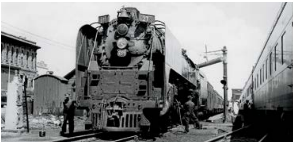
Northern 827 on the westbound Overland has her rods greased and tender filled with water at Rawlins, Wyo., on August 17, 1951. The eastbound Idahoan loads at right.
