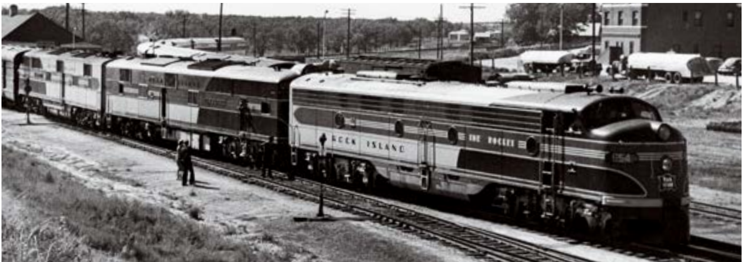
4 /// The E8A from Denver backs onto the Springs section's locomotives. The AB6 was custom-designed with a flat front to give the combined train's power a symmetrical A-B-A appearance. All photos are from September 14, 1952.
