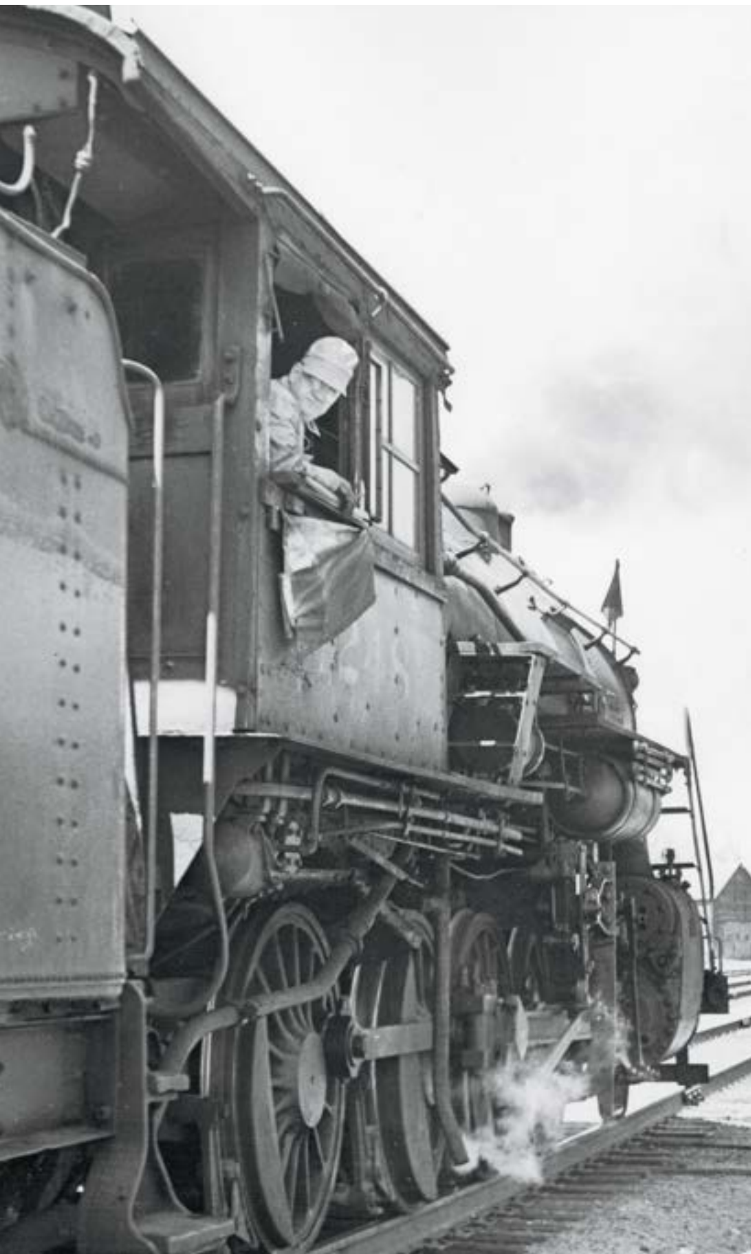
Engineer John Wilkins looks down from the cab of locomotive 1248 as the way freight makes another move. The 2-8-0 was built in 1913 by the road's West Milwaukee Shops.
