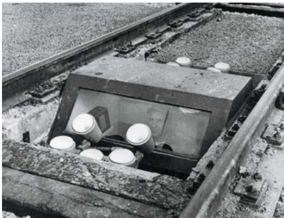
From between the rails, an inspector watches for problems on the undersides of cars. Chesapeake & Ohio
