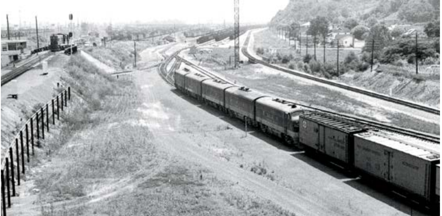
Two Baldwin road-switchers wait on Fitzpatrick's hump before classifying Second 95's cars while five F7s arrive with train 92 from Cincinnati. This view is from the control tower; the line to the right of the light tower takes passenger trains around the yard.
