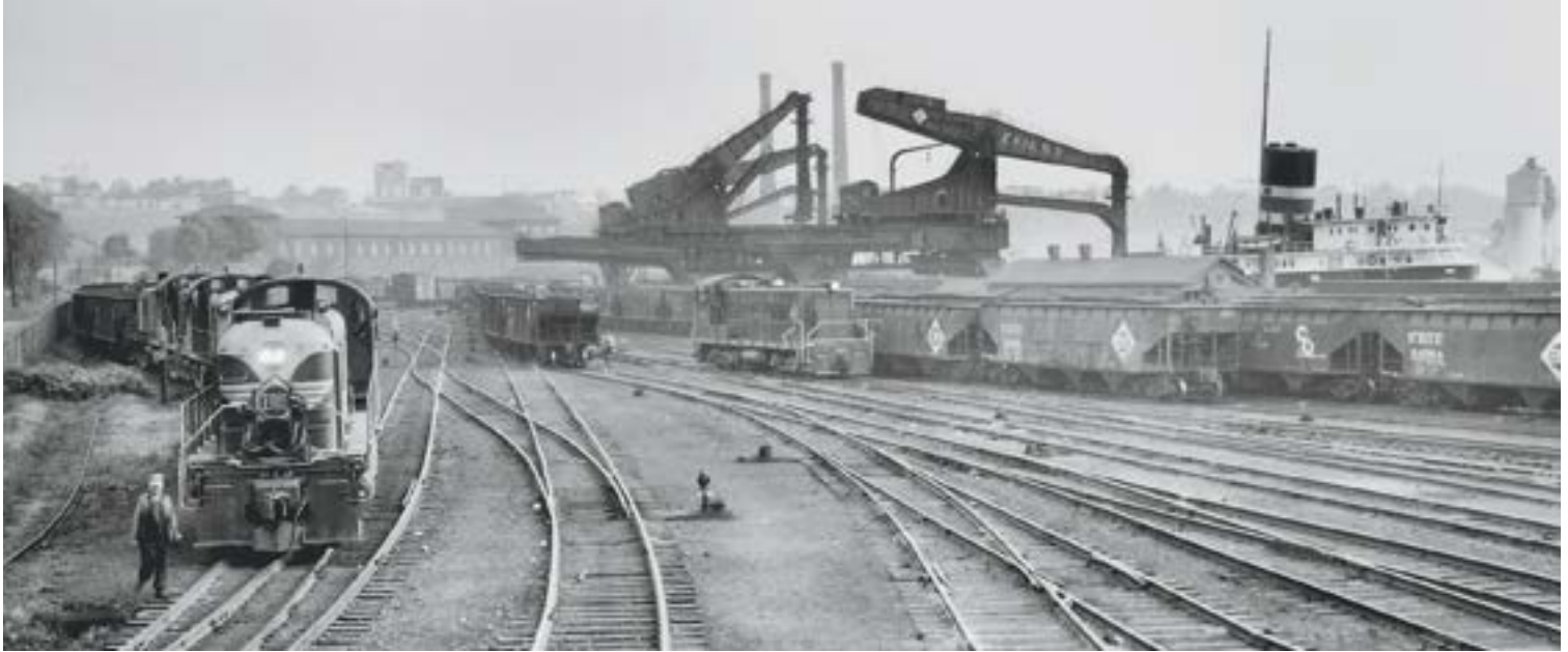
Hulett's unload a lakeboat as RS3s prepare to depart and a Baldwin switcher scurries about at the Erie's Cleveland ore dock in 1960.
