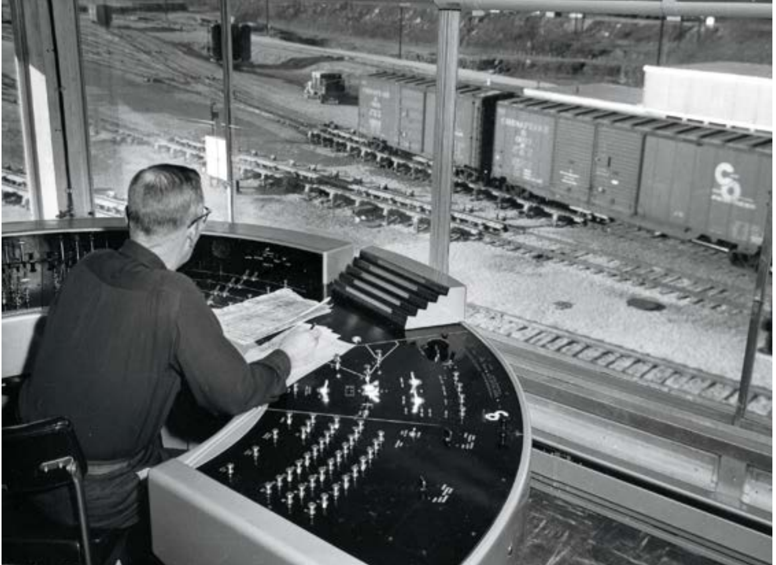
In a view from Fitzpatrick's control tower, boxcars pass over one of the yard's four group retarders; beyond the cars is the signal maintenance shop. Fitzpatrick opened in 1959, at the height of the "push-button" yard era. Note the C&O emblem on the console. Chesapeake & Ohio
