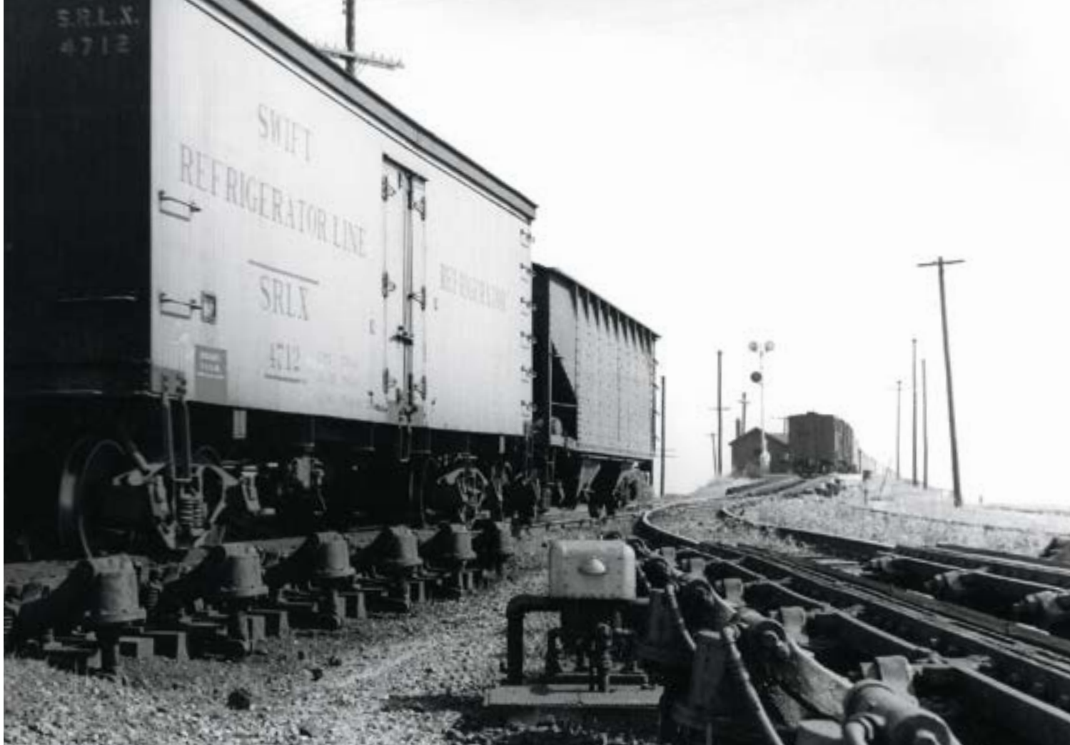
A few years after Galesburg Yard's completion, freight cars crest the hump and then are slowed by the master and group retarders.
