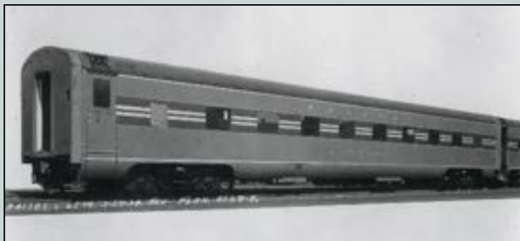
CITY OF TOLEDO: 17-roomette sleeper (plus one section for porter); two per typical consist; 10 built; City of -series names.
