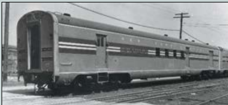
NO. 5020: Mail-baggage car with 60-foot Railway Post Office section; one car per typical consist; 4 built; Nos. 5020–5023.
