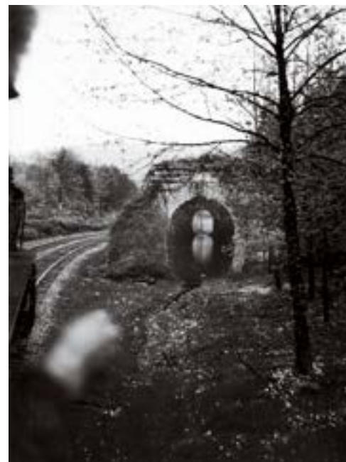
West of Chattanooga, a view from the engineer's side of a locomotive cab shows a pre-Civil War tunnel, long since bypassed by the NC&StL's double-track main line.
