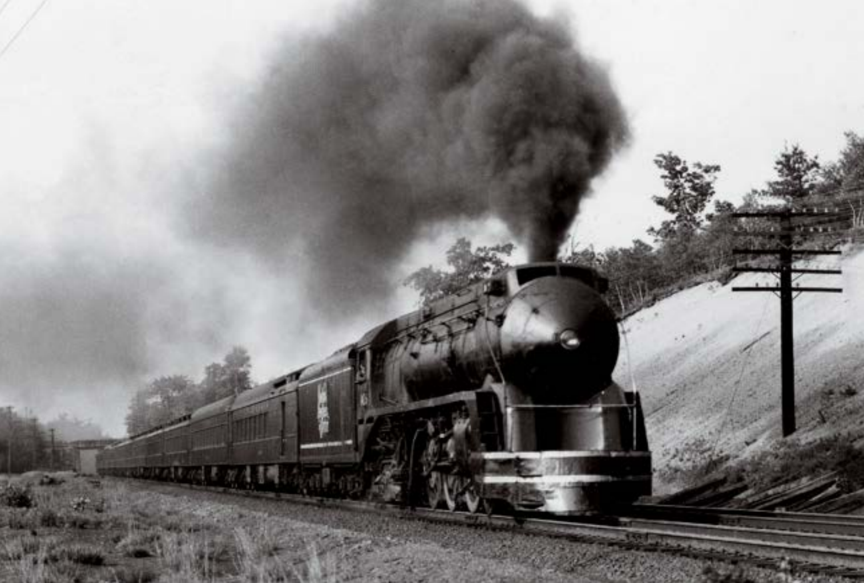
For a few years in the late '30s, the steam queens of NH's Shore Line were 10 class I-5 4-6-4s. The handsome Hudsons' wheel-balance woes prompted NH to begin acquiring a fleet of 60 DL109 diesels in 1941. Here, an I-5 roars west with the Merchants at Sharon, Mass.
