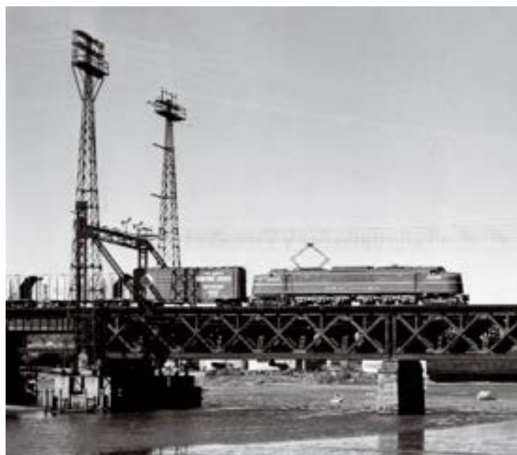
In another view at Cos Cob, a freight crosses the Mianus River on a bridge that includes a gap in the catenary above the draw span. This is one of a dozen drawbridges on NH's Shore Line.
