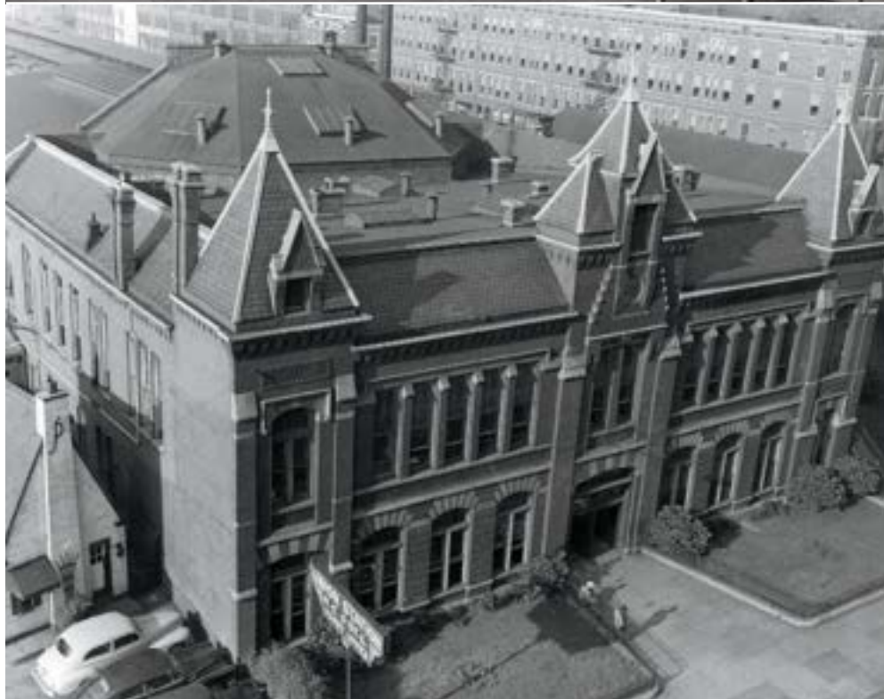
Civil War history is on view at Chattanooga Union Station, where in 1891 the NC&StL placed on display the General (top), the 4-4-0 that led the "Great Locomotive Chase" of 1862. The terminal opened in 1858; the headhouse (above) was built in 1881-82.
