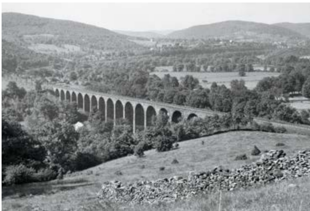
The famous Starrucca Viaduct, a landmark on the Erie Limited 's route at Lanesboro, Pa., was observing its centennial year at the time of this June 17, 1948, photo. The great stone bridge measures 1,040 feet long and stands 100 feet above Starrucca Creek.
