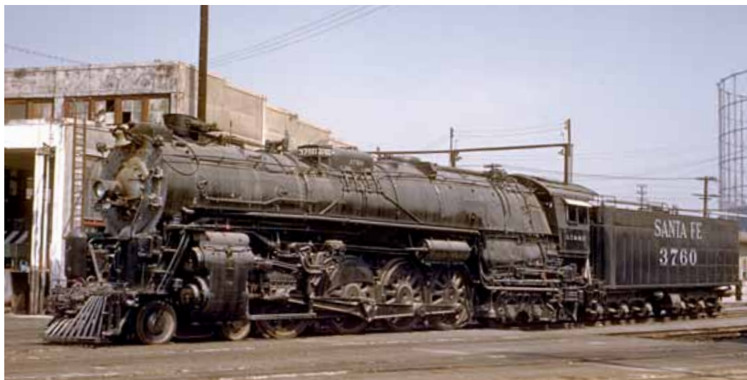
Santa Fe 3760 (above) shows the effects of the late-1930s rebuilding of the 3751-class 4-8-4's; pictured at Los Angeles on August 21, 1956, it had been stored for two years. Engine 3782 (right) of the 3776 class crosses the Arroyo Seco Parkway as it climbs from L.A. to Pasadena with the Chief ; it's 1946, but 3782 still wears its wartime headlight visor.
