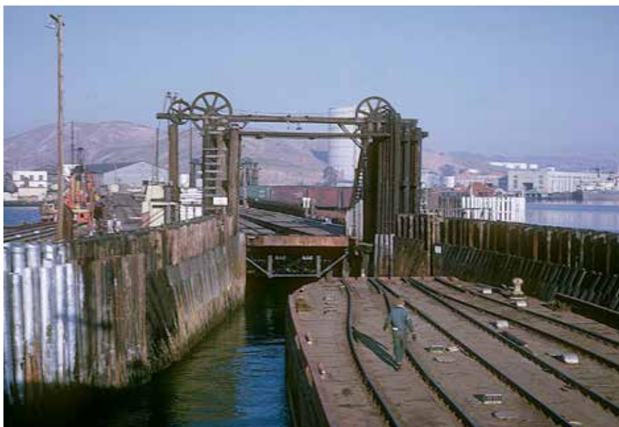
Although taken at Ferry Point in 1962, this photo shows the same kind of apron hoist used at Alice Street, and the three tracks on the car float squeezing together to meet the closely spaced tracks on the apron. Jack Whitmeyer photo
