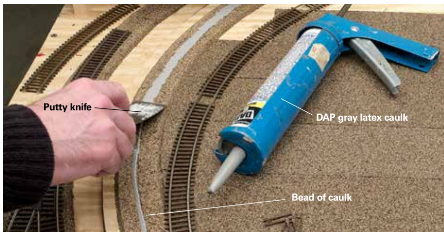
Fig. 4 Caulk. David used gray DAP caulk to attach the track to the roadbed. After laying a bead of caulk on the cork, he smoothed it with a putty knife.
