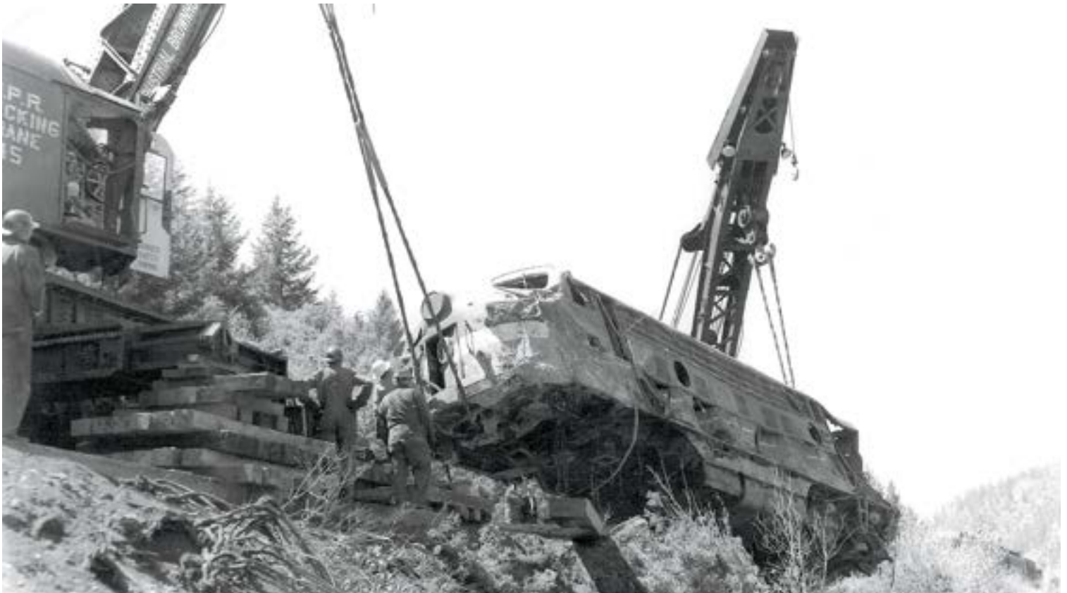
Two days after it flew off the track at 87 mph, third unit F9A 6701C is lifted back onto the right of way by NP derricks 45 (left, from Spokane) and 47 (Missoula). All 4 locomotives and 17 cars involved in the Evaro derailment were repaired and returned to service.
