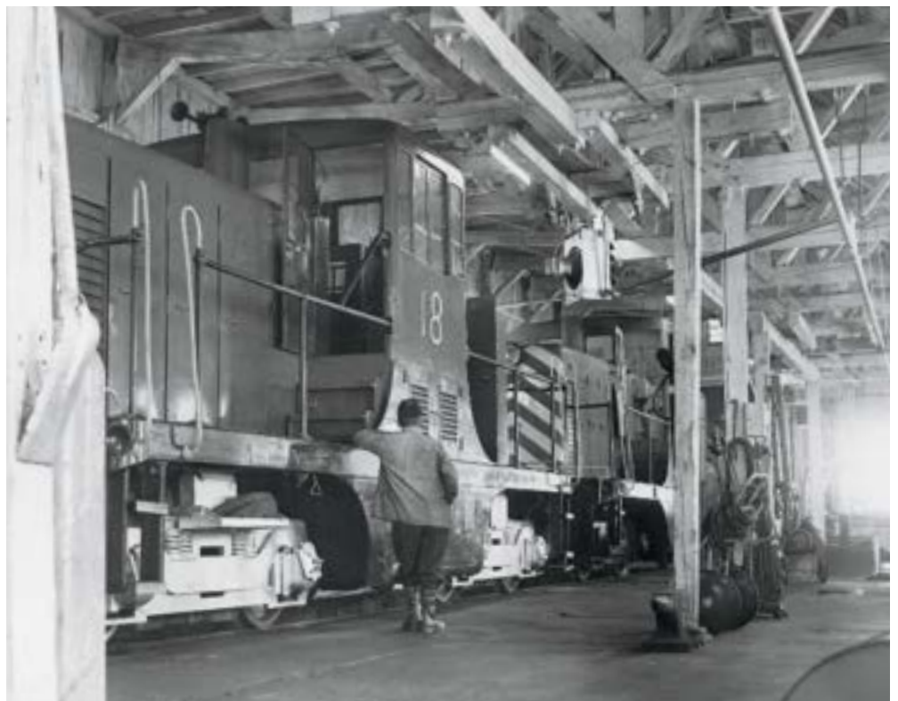
HT&W's entire locomotive fleet of two red 44-tonners enjoys the shelter of the Readsboro enginehouse in January '62. No. 18 is ex-B&M, while 16 came from Maine pike Sanford & Eastern, a sister to HT&W in the Pinsly-owned family of short lines.
