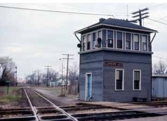
At the Lapeer Junction tower (pictured in 1972, looking south), we were instructed by our Superintendent on how to proceed.
