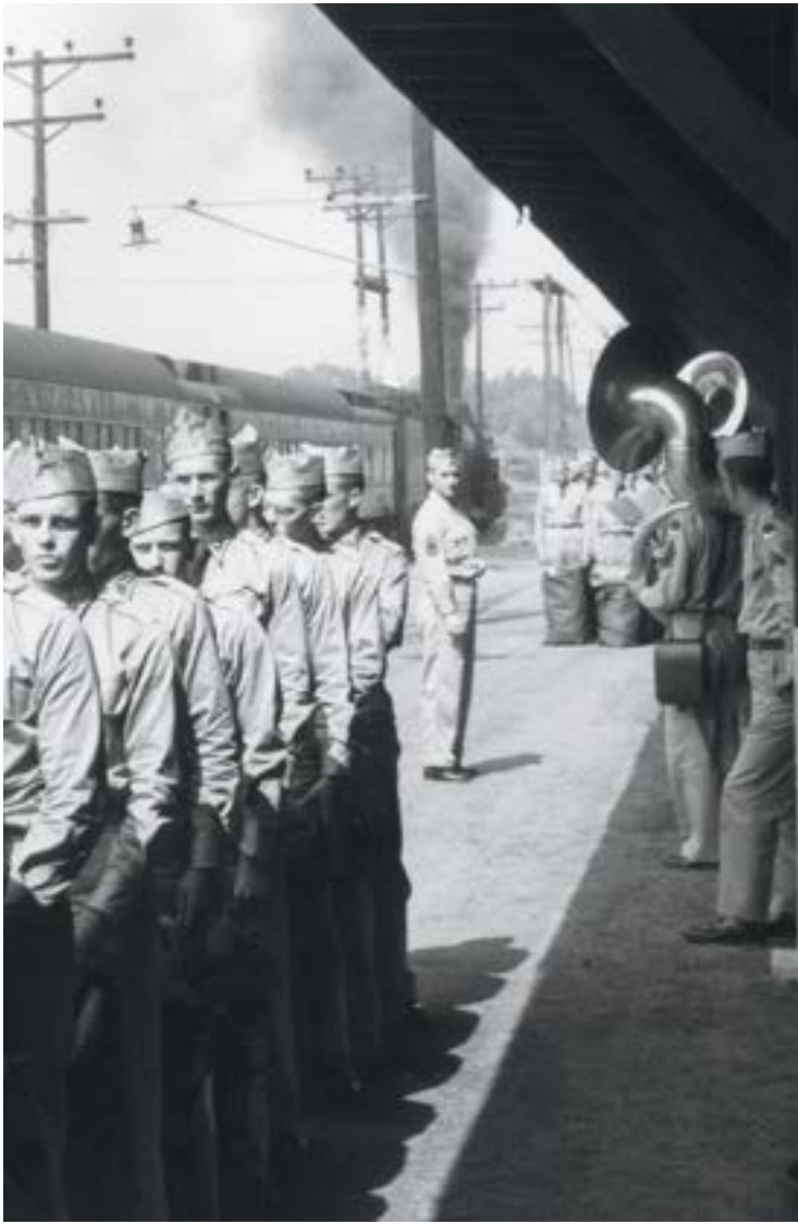
Each busload is assigned to a particular Pullman car. On leaving the buses, the men line up in columns of twos. After the buses pull out, the troops file aboard the cars, to the accompaniment of a military band. Beyond, 5040's fireman gets his fire ready.
