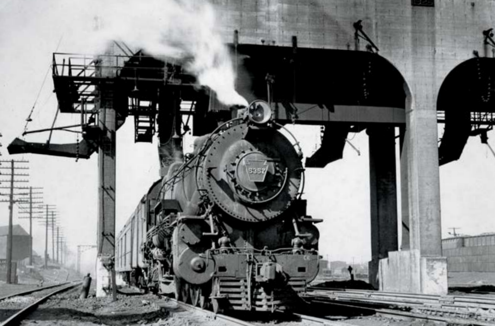
K4s 5357, still with old-style headlight and pilot, takes fuel at the mainline coal dock just east of Fort Wayne before continuing east.
