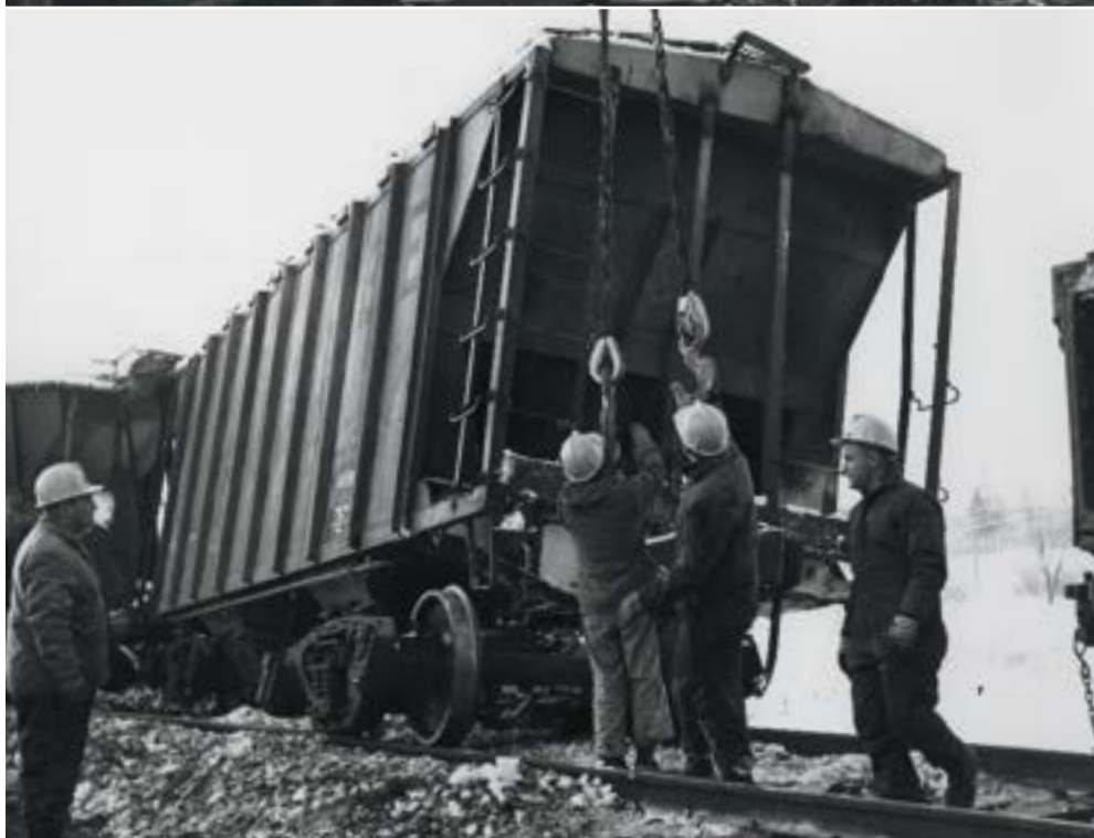
GTW's 200-ton crane 50007 gingerly lifts a derailed Milwaukee Road covered hopper back to the rails (top), and carmen of the Durand Auxiliary crew put their skills and nerve to work to assist (above), as clean-up of the 41-car derailment of eastbound train 812 at the "PO&N bridge" at Imlay City, Mich., progresses in the early morning of April 3, 1970.
