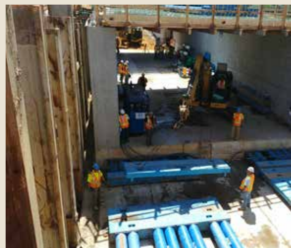
The Covert Avenue underpass in New Hyde Park, N.Y., is jacked into place on Aug. 24, 2019. The jacks are at the edge of the concrete box in the foreground. MTA
