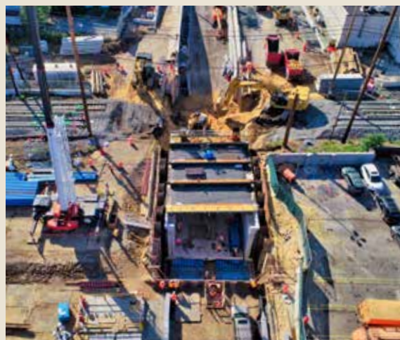
An aerial view shows the concrete box and bridge for the School Street underpass, completed and ready to be moved into place via box jacking, on Oct. 4, 2020. MTA
