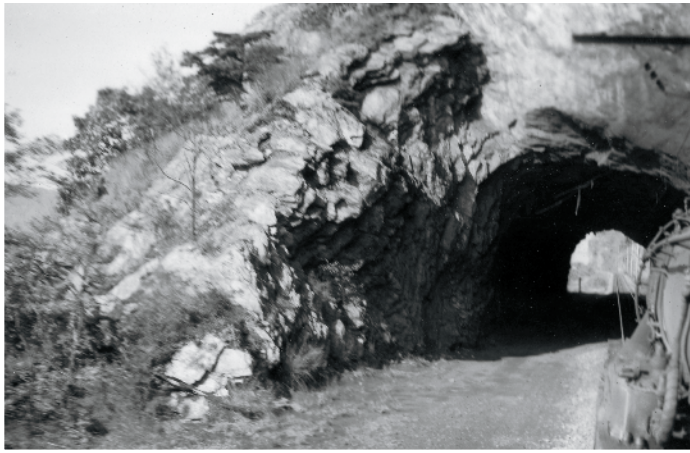
The train enters Wildcat Tunnel. There are three such bores — Wildcat, Williams, and Frazer — and they're really only holes blasted through huge rocks.
