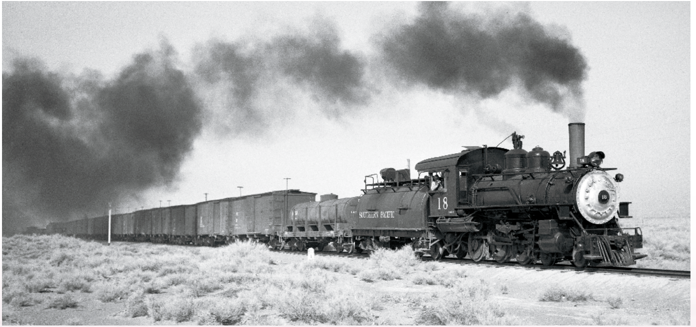
Southern Pacific Ten Wheeler No. 18, trailing its familiar water car, rumbles along the south end of the railroad's narrow-gauge near the town of Mount Whitney, Calif. Much of the equipment in this 1951 photograph was already more than 50 years old. Walter H. Vielbaum
