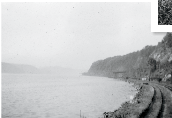
West of Harbor, two of the overhead water drainage chutes are visible. They help direct water off the railroad right-of-way.
