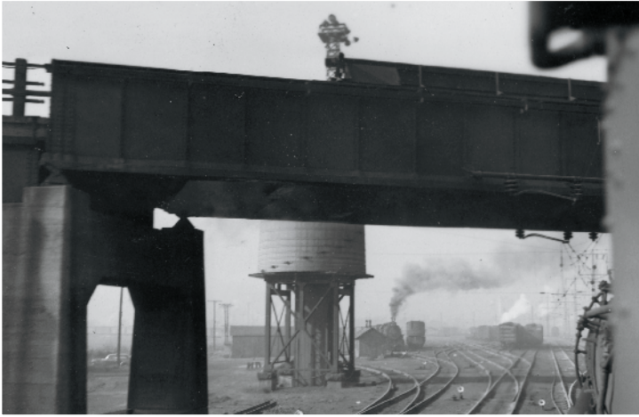
Running the northbound track, the train eases into the yard at the north end to pick up at Edge Moor.
