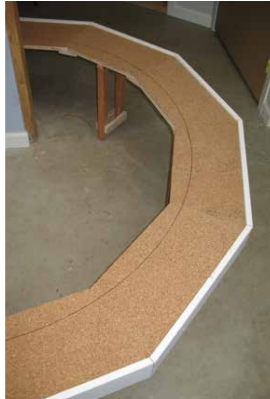
2 On-site assembly. The trapezoid panels were delivered to Dave's basement for final assembly. He added cork sheet on top of the plywood before installing the track.
