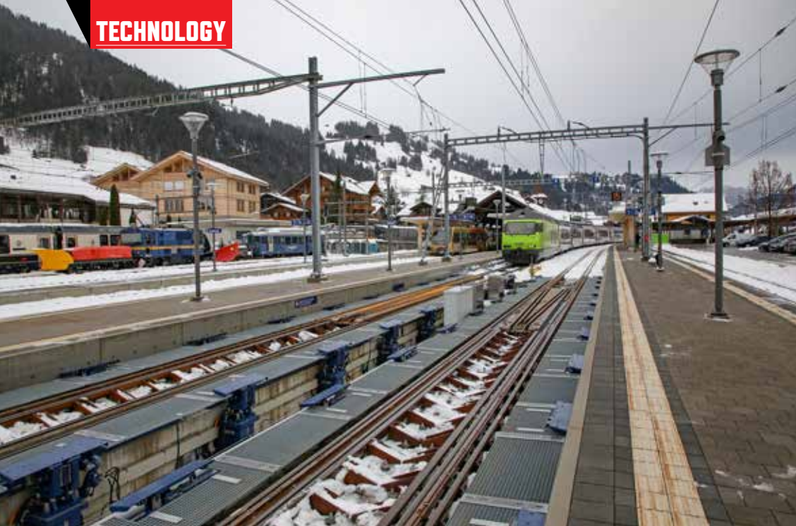
The gauge-changing equipment at Zweisimmen. The GPX train, with a bright green BLS standard-gauge locomotive at the rear, has already undergone its conversion. Trains are always moved through the equipment by MOB's meter-gauge locomotive. Two photos, Keith Fender
