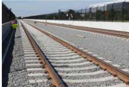
Newly laid rails on concrete ties stretch into the distance during construction of the Silver Line of the Washington, D.C., Metro system in September 2018. Though some railroads and routes have concrete ties, most tracks in the U.S. still have wood ties. Sol Tucker photo
