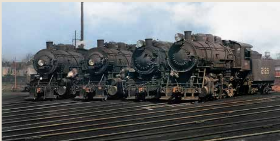
Products of the L&N's South Louisville Shops (from left): Nos. 1303 and 1291, both class H-8 2-8-0s built in 1911, No. 2149, a member of the C-2 class 0-8-0s constructed between 1922 and 1925, and No. 2125, a C-1 class 0-8-0 completed in 1923. No. 2132 is from this same class.
