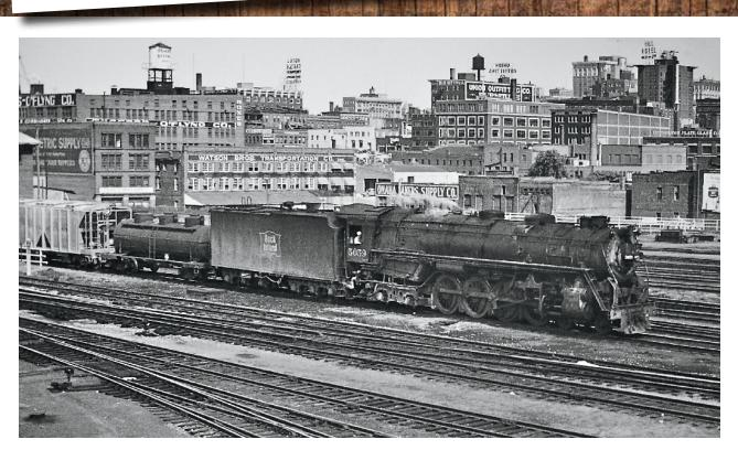
Eastbound Rock Island 4-8-4 No. 5059 moves through the maze of trackage west of the Omaha station with a freight train. The 4-8-4-type was the largest steam locomotive on the Rock's roster, classed R-67B and carrying Nos. 5000-5064 and 5100-5119.
