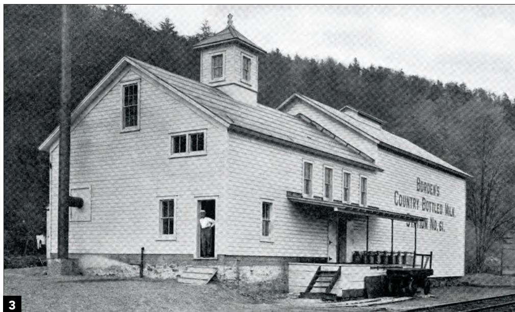
Borden had receiving stations and bottling plants in many locations. This one is at Cohecton, N.Y., on the Erie. It's a two-story wood structure with large adjoining ice house at right. Jeff Wilson collection
