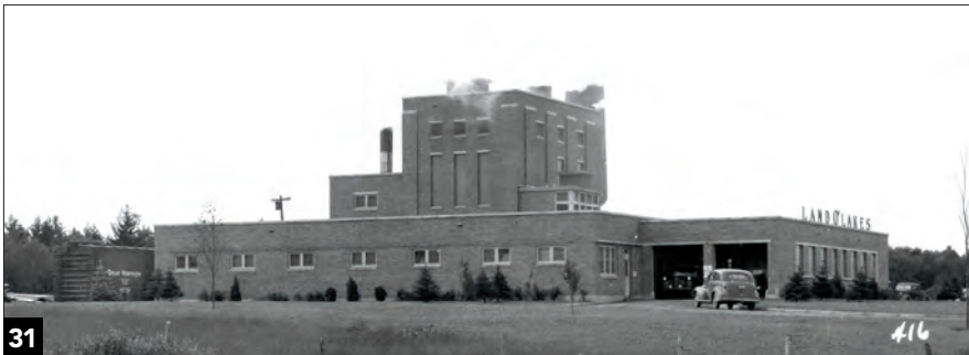
31 The Land O'Lakes dried milk plant at Sebeka, Minn., had a rail spur on the Great Northern (note boxcar on left). Bulk milk trucks were unloaded under cover at right. Jeff Wilson collection
