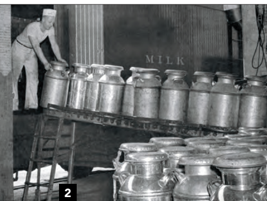
A worker unloads a milk can car, placing cans on a portable gravity conveyor at a milk plant. Each car typically held between 200 and 300 cans, each of which weighed about 113 pounds when full. U.S. Department of Agriculture
