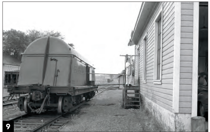
Tank cars were set out the previous day or evening for loading, with precise spotting needed (note the loading pipe). It will be picked up shortly after it's loaded. New York Central
