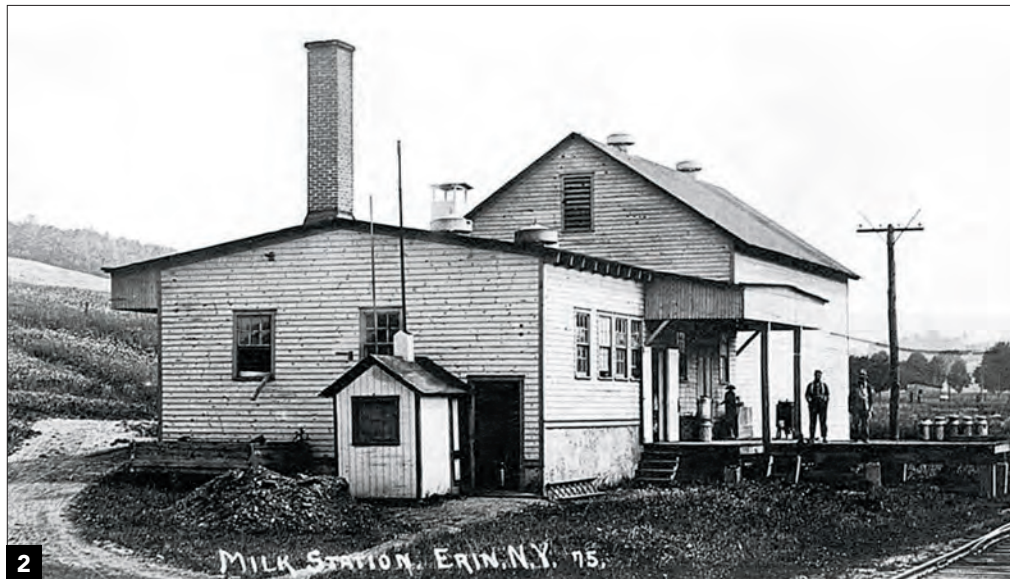
The “creamery” at Erin, N.Y., on the Lehigh Valley, exemplifies the small receiving station. The turn-of-the-century view shows an open platform and the larger icehouse to the rear. Jeff Wilson collection
