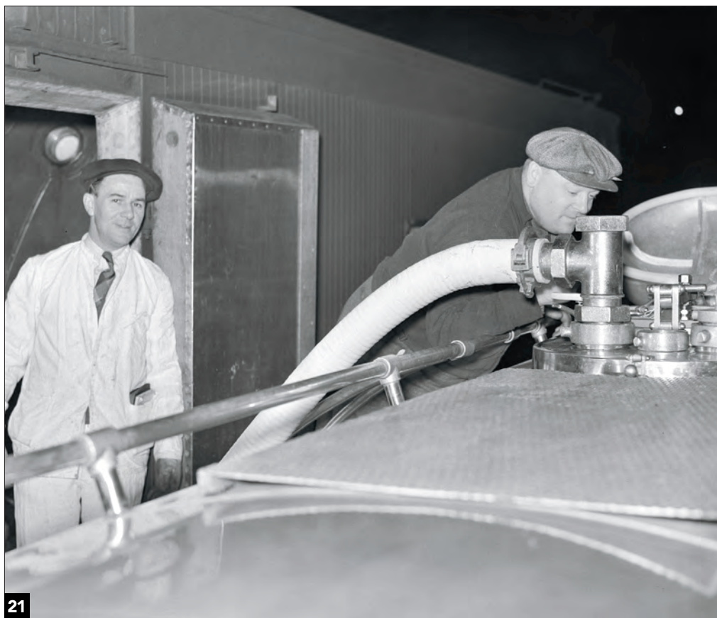
One of the GPEX car's tanks is visible behind the worker at left (an access window is just to the left of his head). The driver has secured the hose to the inlet valve of the truck tank. Arthur Rothstein, Library of Congress
