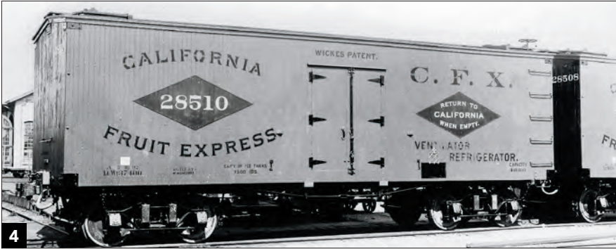
4 This Wickes Patent refrigerator car was state-of-the-art when built in 1892. It's an all wood (truss-rod underframe) 32-foot car with ice bunkers at each end. It's not equipped for high-speed service, and rides on standard archbar trucks. Most reefers of the period were in meat or vegetable service. Trains magazine collection
