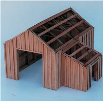
This view shows the crosspieces that will hold the roof.
