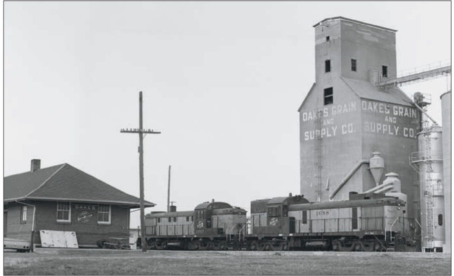
Iconic structures of the American plains include small wood-framed depots and grain elevators (“prairie skyscrapers”). William S. Christopher
