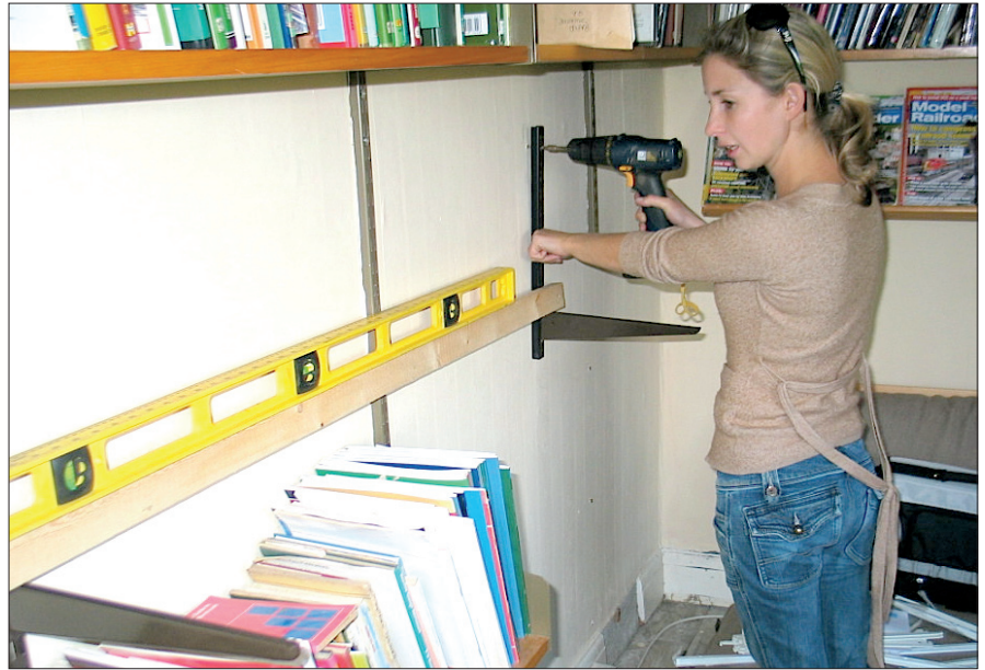
It's vital that the notches in the shelving tracks align in order to keep the shelf level. A straight 1 x 2 or 1 x 3 and a long spirit level work well for this. It helps to have an extra pair of hands (as here those of the author's daughter, Elsa) assisting in the installation process.
