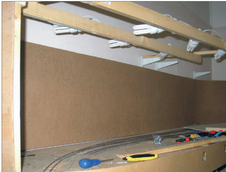
Here's an overhead lighting raft using fluorescent bulbs for a deep-scene shelf layout, supported by shelf tracks. The backdrop is 2mm medium-density fiberboard.
