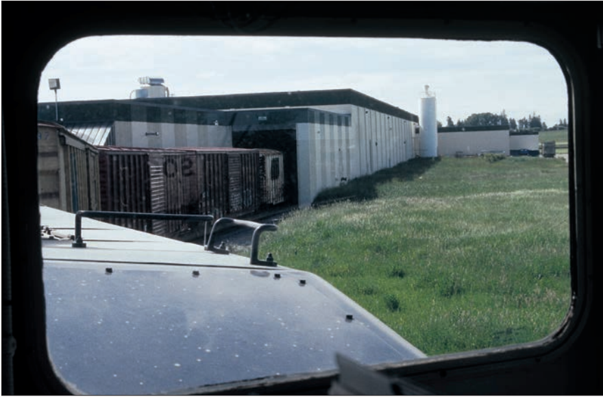
Modern industrial structures, such as this warehouse on Progressive Rail tracks in Lakeville, Minn., are low in height but big on footprint. This leads to sprawling track layouts that call for wider sites. Jim Hediger
