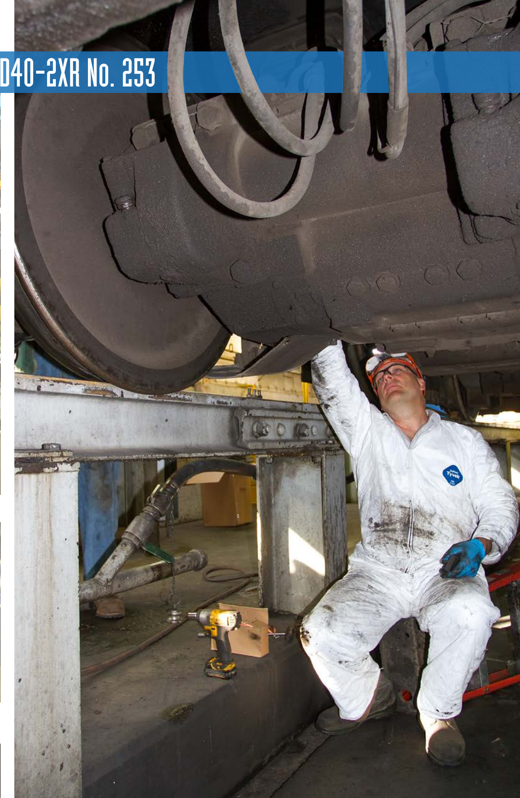
Veteran electrician Steve Howes changes traction motor brushes on No. 253.
