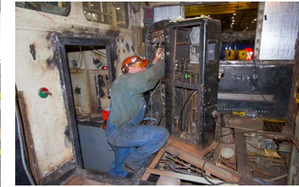
Ben Hampson rewires the control stand of former WC No. 3025.
