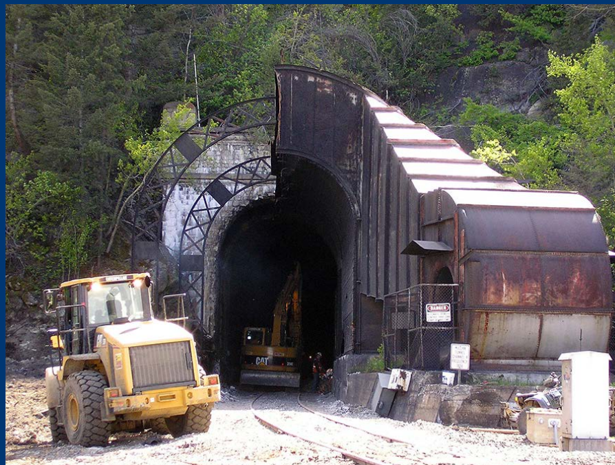
In June 2009, the unique blower system structures at Mullan Tunnel's east portal are being dismantled. Montana Rail Link
