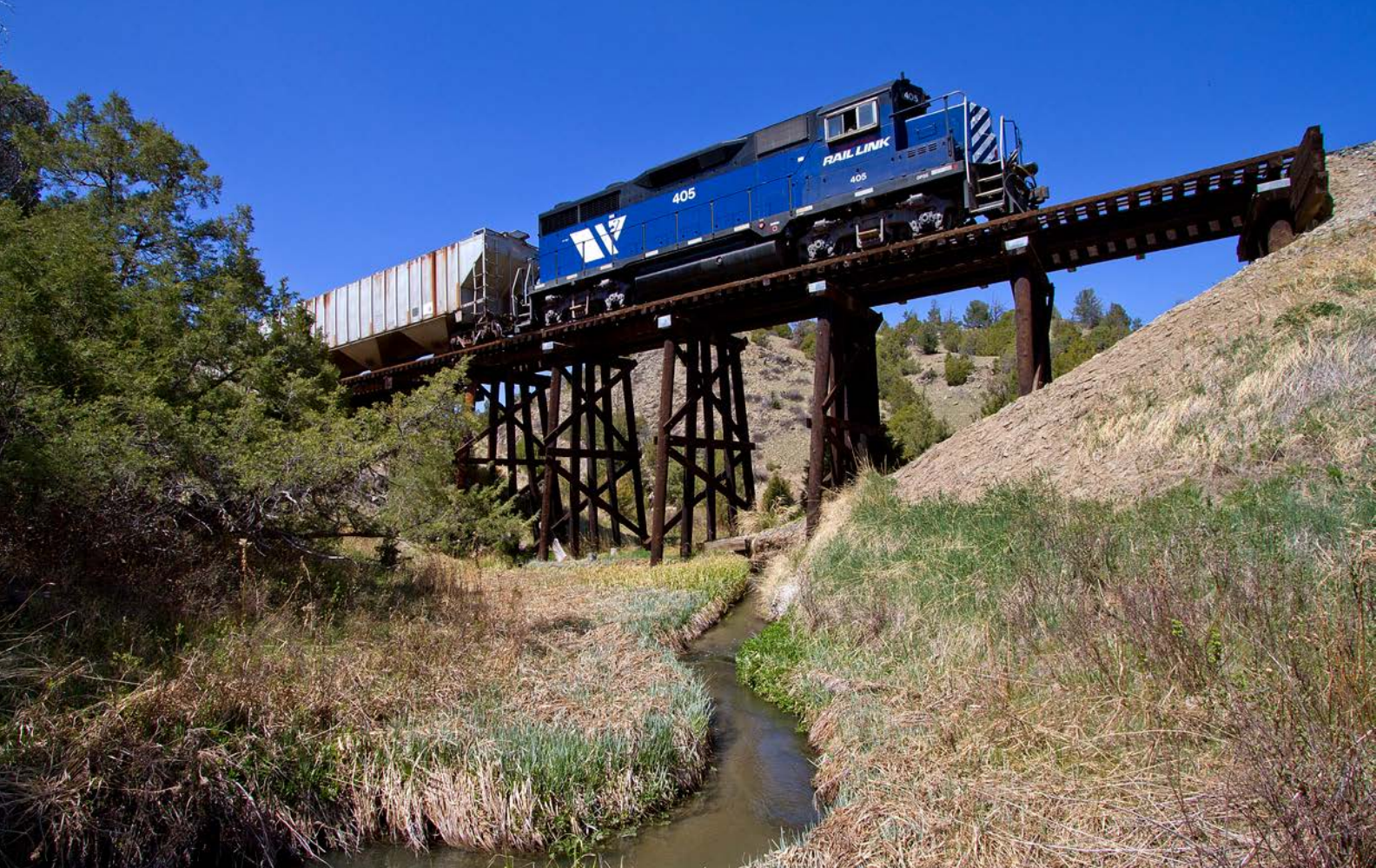
Montana Rail Link's 844 local crosses Little Antelope Creek on an old but well-maintained wood trestle 4 miles north of Harrison, Mont.
