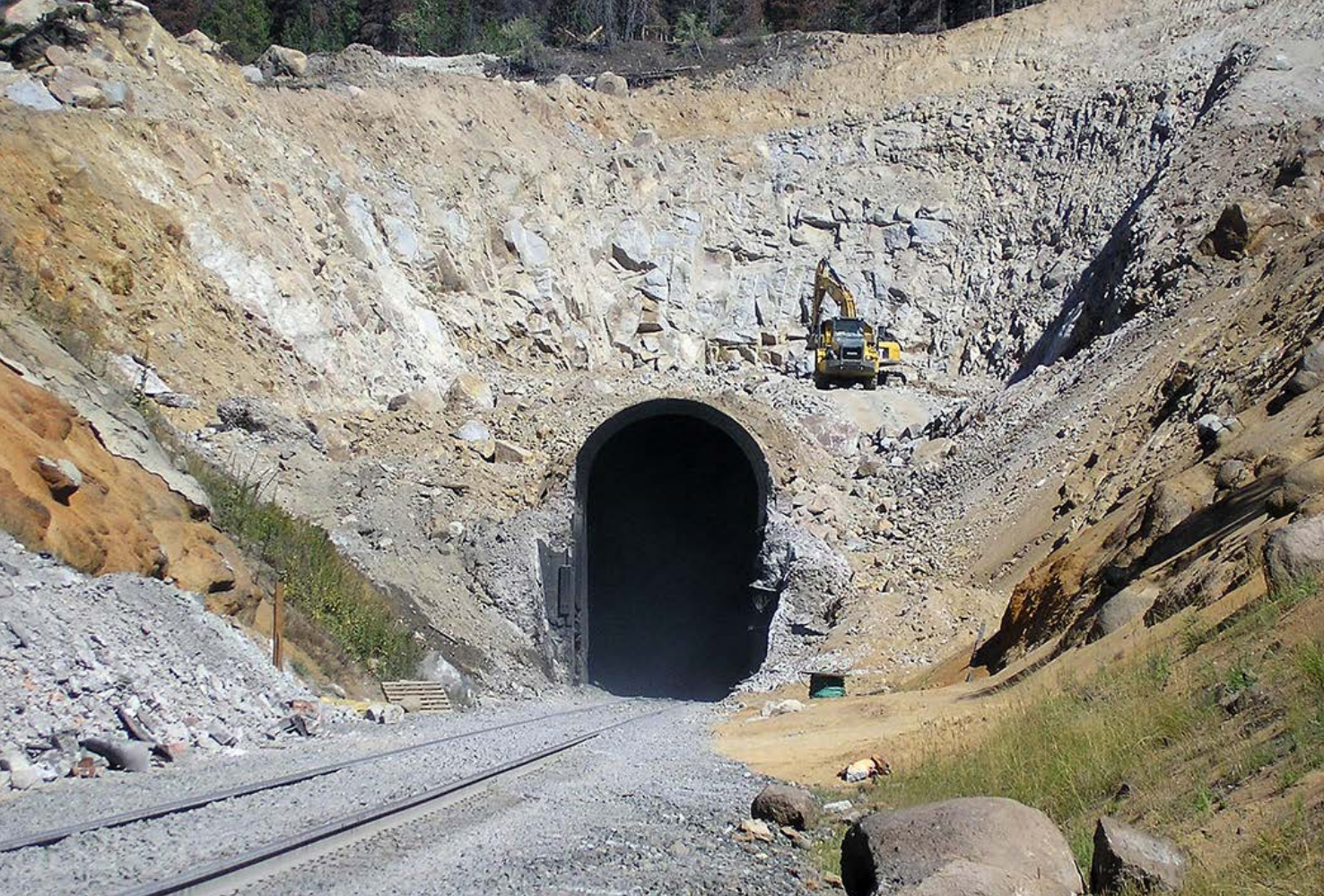
In September 2009, contractors excavate above the west portal of the tunnel, exposing the old brick lining. Montana Rail Link
