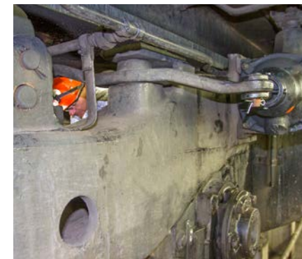
Electrician Steve Howes works in tight confines underneath No. 253.
