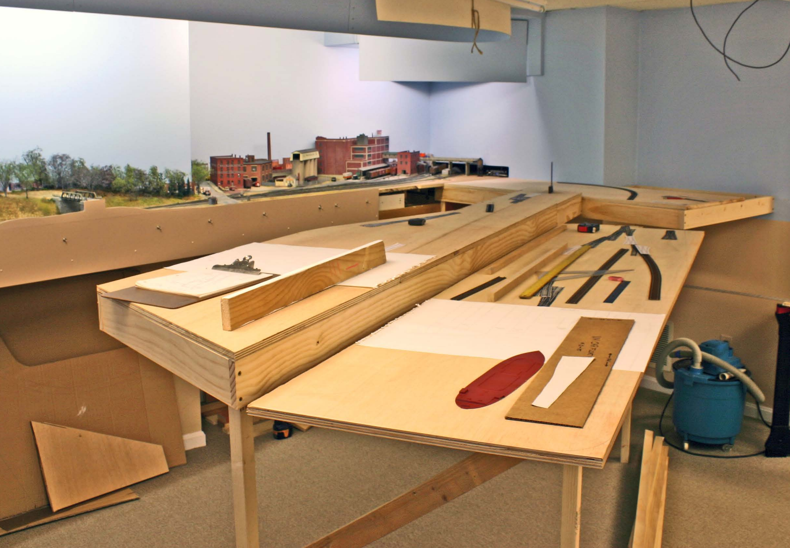
Fig. 1 Early construction. The plywood for one of the two peninsula sections has been mounted on the grid. In the foreground, cutouts of the car float barge and tug are used to determine position before attaching the plywood.
