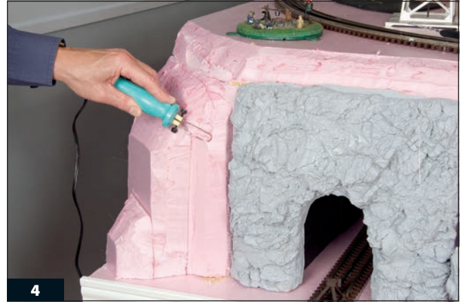
4 After installing pieces of 2" foam board around the portal, use a hot wire cutter to carve a gradually sloping face.
