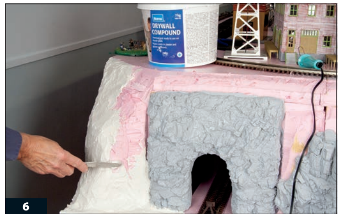
6 Cover all exposed surfaces of the hillside with drywall compound and fill the seams between the foam boards and the portal.
