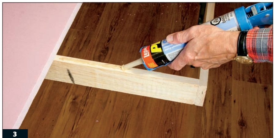
To apply the adhesive, draw a bead of cement along the wooden frame and then press the foam board in place on top of it. Then remove the foam board to spread the adhesive and reset it.
