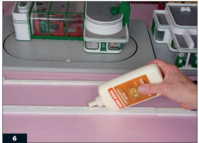
Cut strips of scrap foam core board to use as shims to raise the streets to the level of accessory bases.
