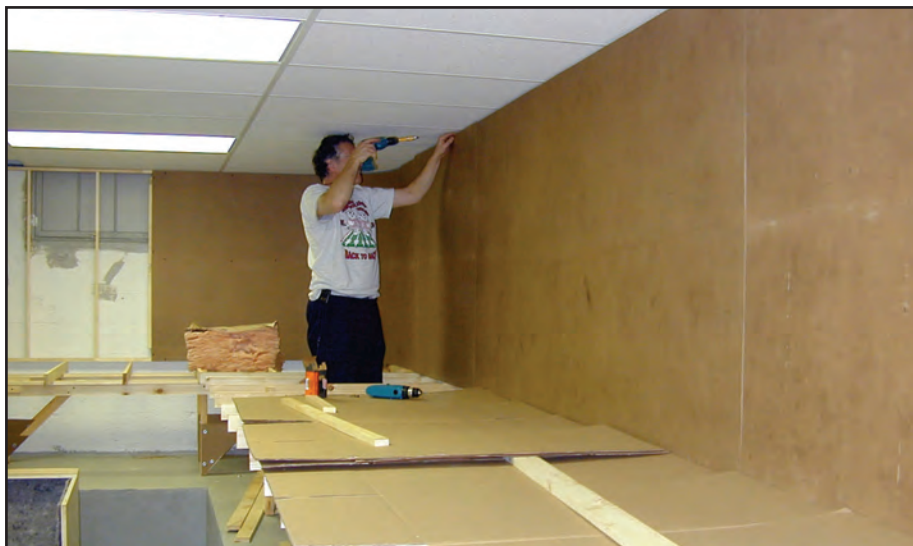
This fiberboard backdrop was mounted on a frame made from 1" strapping. The seams will be taped and spackled. Don Holloway layout
