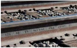
Newly installed rail on CSX's Toledo Subdivision near Deshler, Ohio, is seen on Oct. 8, 2010. The first part of the manufacturer's marks on the side of the rail, 136 RE, identify this as 136-pound rail, typical of modern main lines. Eric Powell photo
