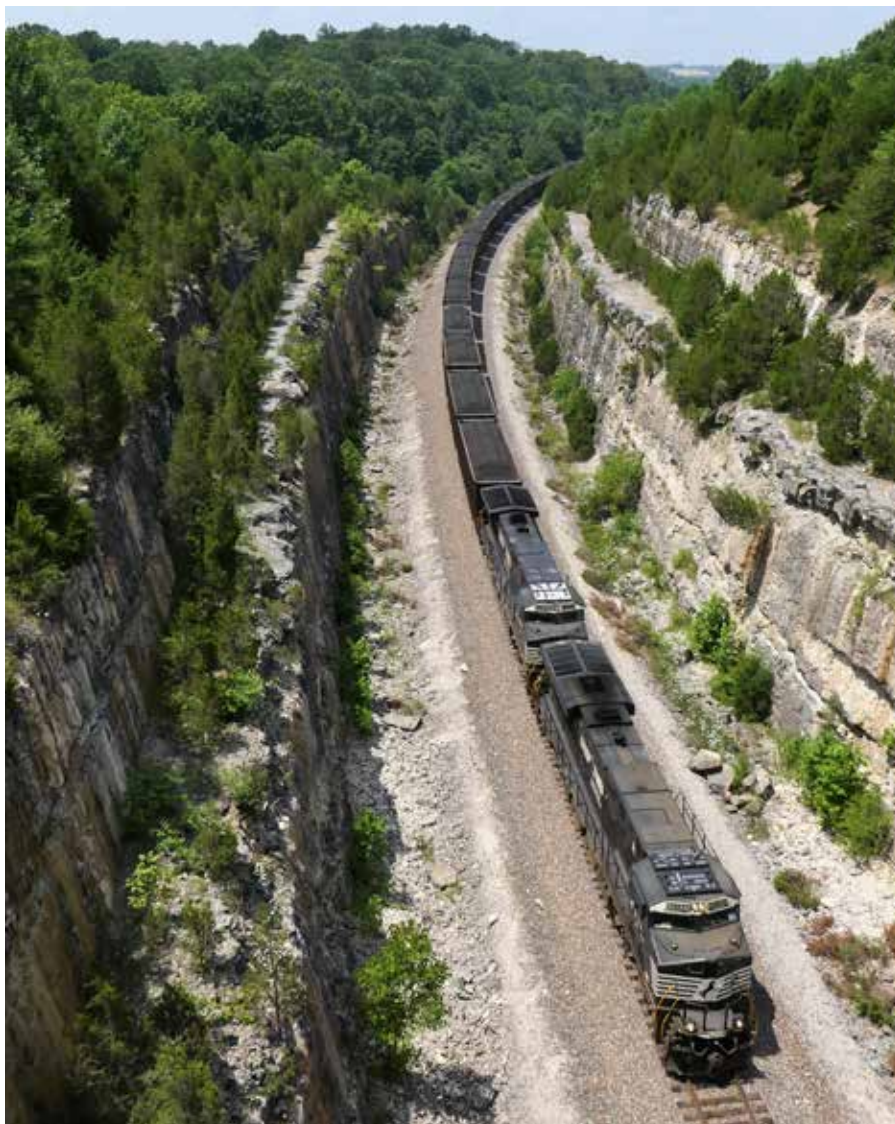
An eastbound coal train navigates a deep rock cut under Tunnel Hill Road Bridge east of Depauw, Ind. The former Southern Railway route links Louisville, Ky., and St. Louis, Mo.
