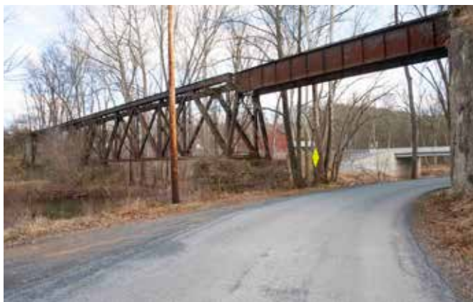
The 275-foot Pogue bridge, located 3 miles south of Rockhill Furnace, Pa., was found to be in good condition after inspection. Dan Cupper
