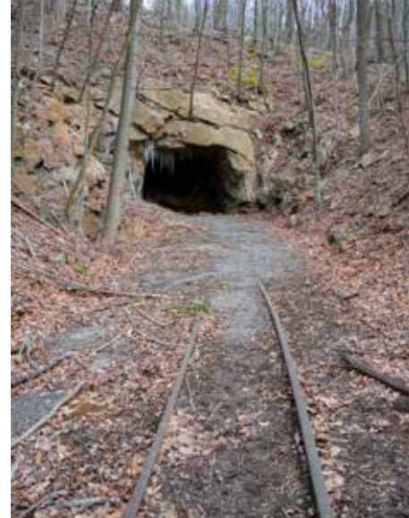
South portal of EBT's Sideling Hill Tunnel, which would be reopened to provide access to the Joller Branch. Dan Cupper
