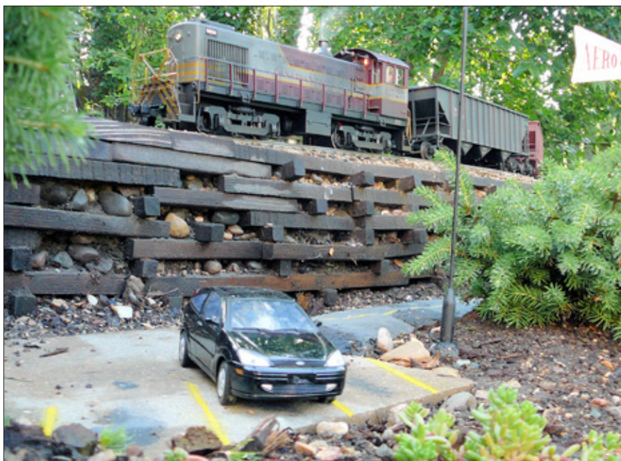
6. An Alco S-4 trundles past on top of the retaining wall, which overlooks the picnic-site parking lot. The color of the cedar cribbing reflects the author's wood preservative, a 50:50 mixture of Minwax dark walnut oil-based stain and boiled linseed oil. A bird's nest spruce partially obscures the cribbing on the right.
