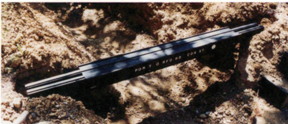
The finished bridge, temporarily in place, still lacks abutments.
