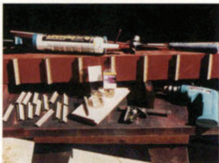
The T-braces were cut from tongue-and-groove flooring. Then they were glued and nailed to the sides of the bridge.
